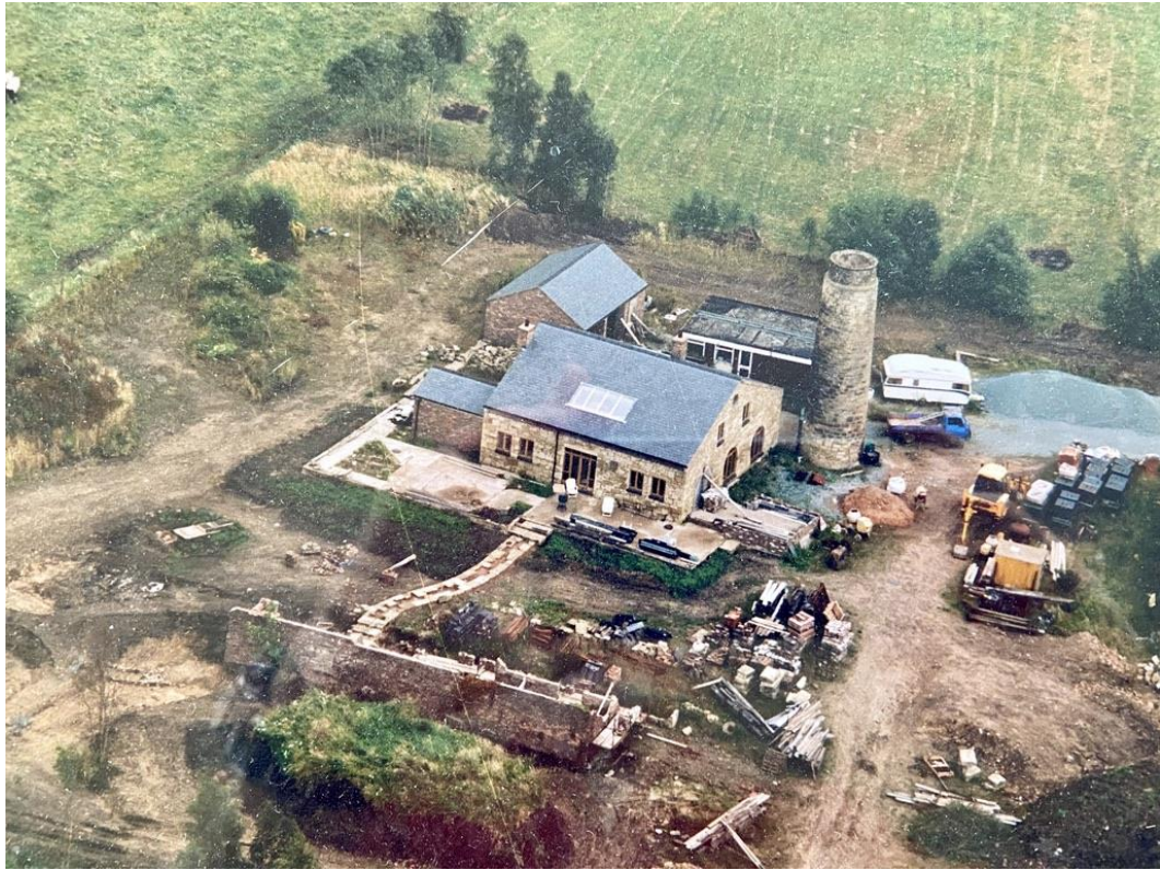
Photo 6 – The beginning of restoration showing the relationship of the main Foundry building, the stone chimney, and the remnants of the former storage building
