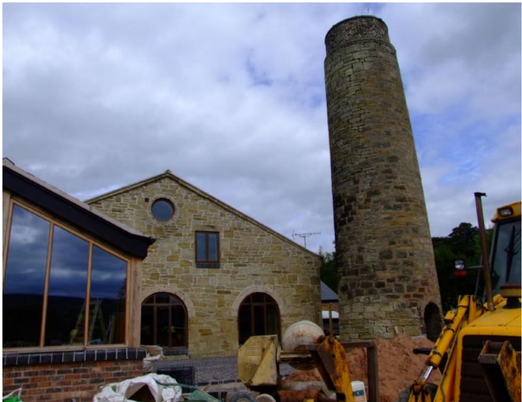
Photo 5 – Work on restoring Pentre Saeson Foundry building
