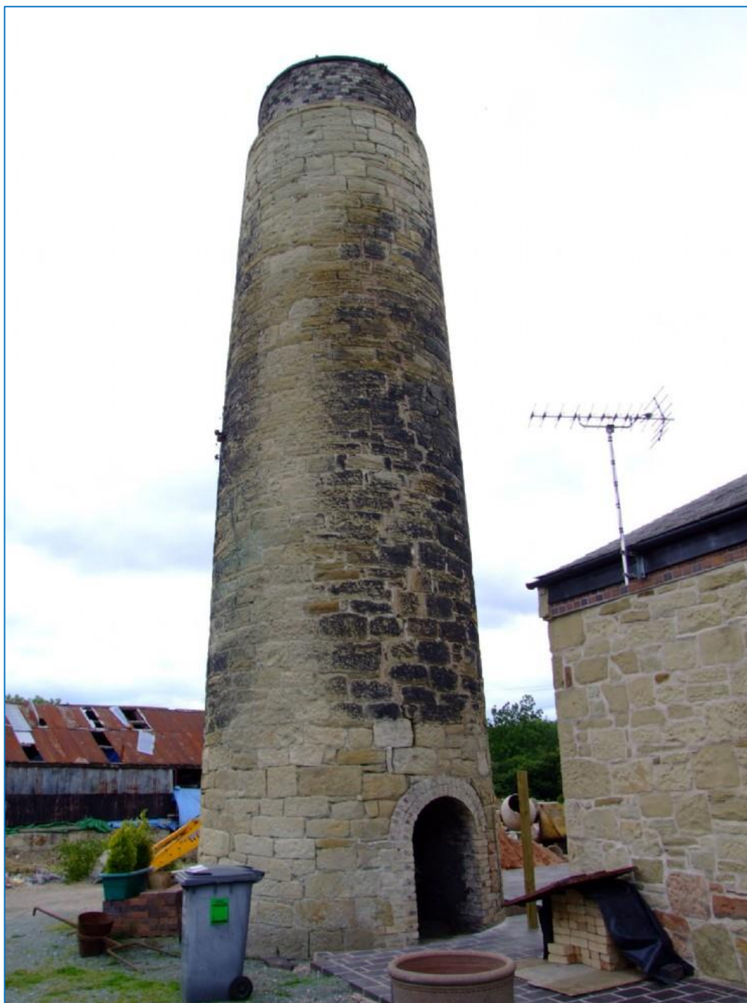
Photo 5 - Pentre Saeson Foundry Stone Chimney
