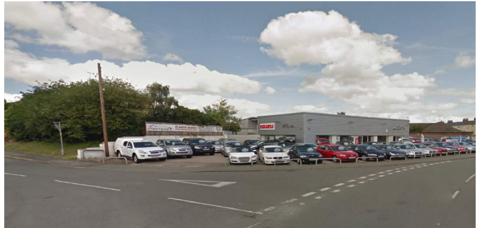
Local commercial car dealership: Aluminium cladding
