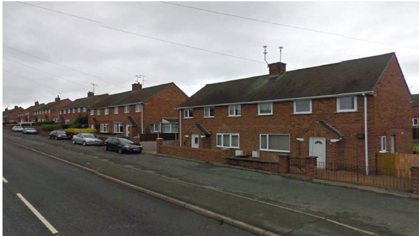
Site Image: residential housing parallel to the site.
