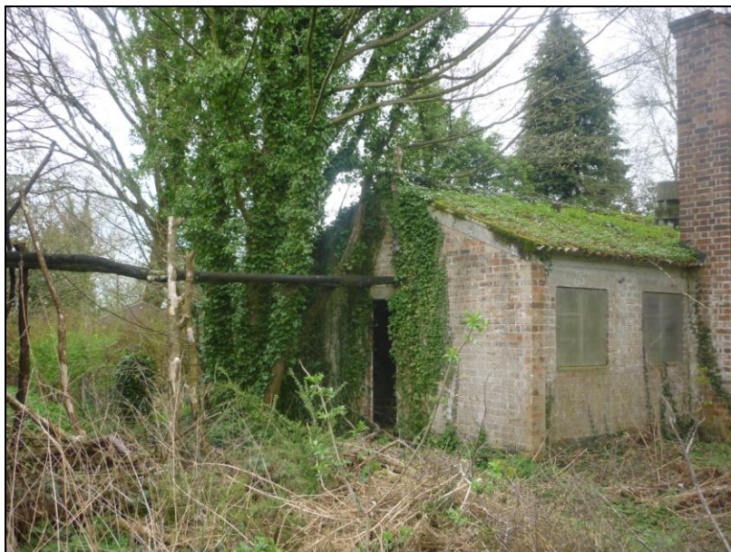
Photo 6 - Trees within G3 abut the various semi-derelict buildings
