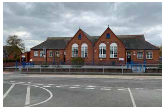
View of the North elevation of the original school building from Bangor Road
