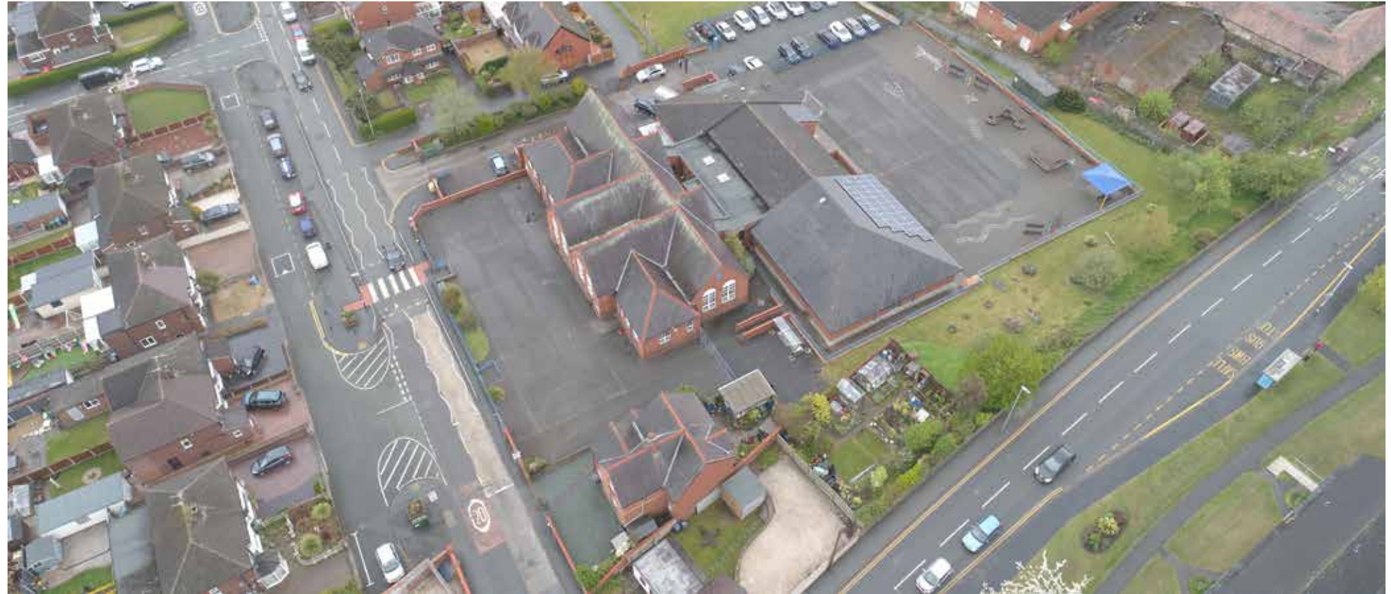
Drone image illustrating the roofscape of the existing building, indicating the numerous extensions the school has previously undertaken
