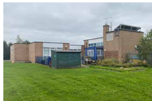
View of the rear elevation from the school playing fields
