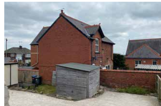
View of the side and rear elevations taken from Ruabon Road
