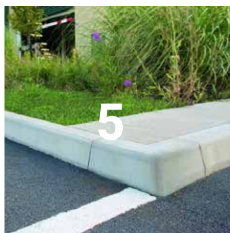
Concrete road kerb & tarmac
