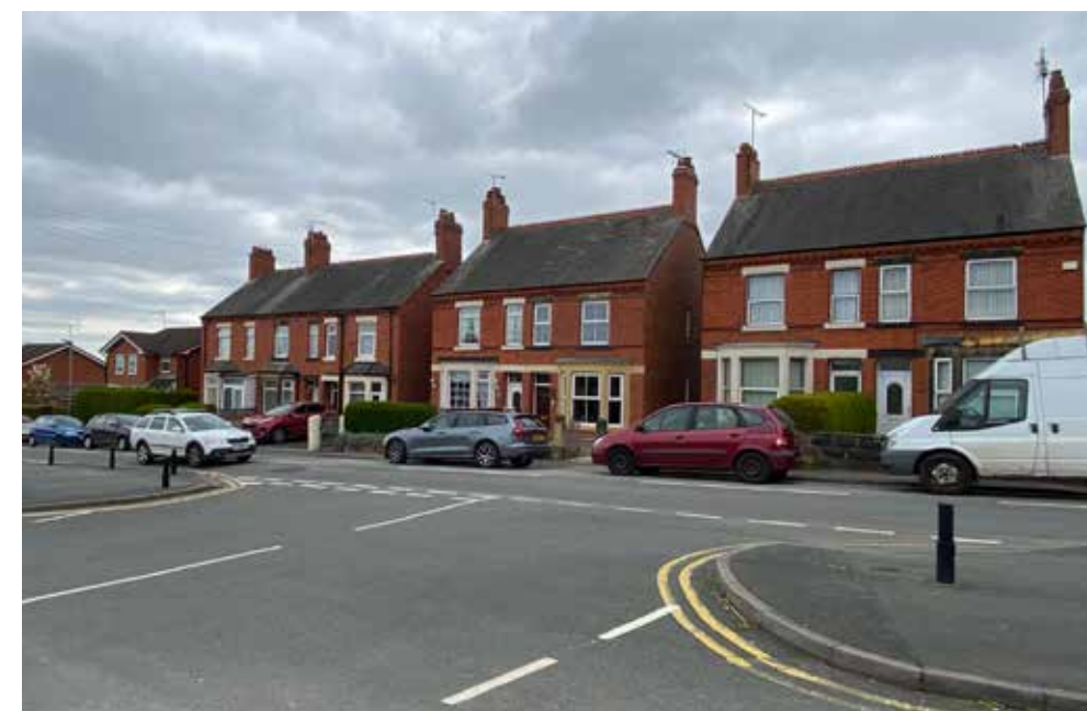
View along Bangor road illustrating the immediate two storey residential context backing onto the school field
