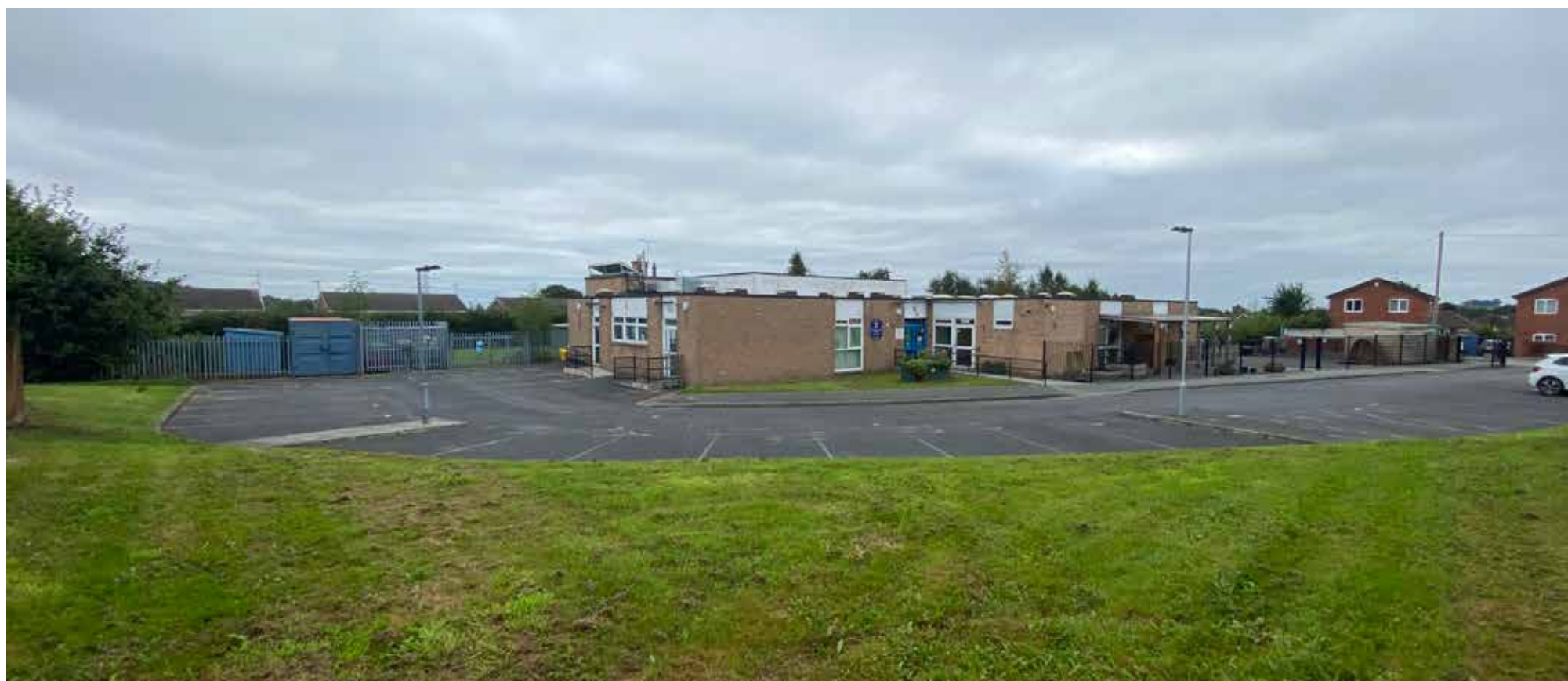
View towards the Main School entrance across the car park
