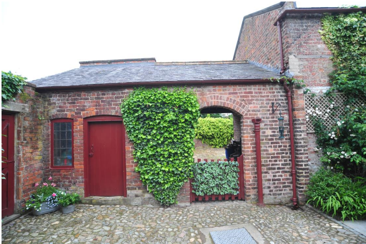
Pl.10: The north wall of the single storey portion of the stable court.
