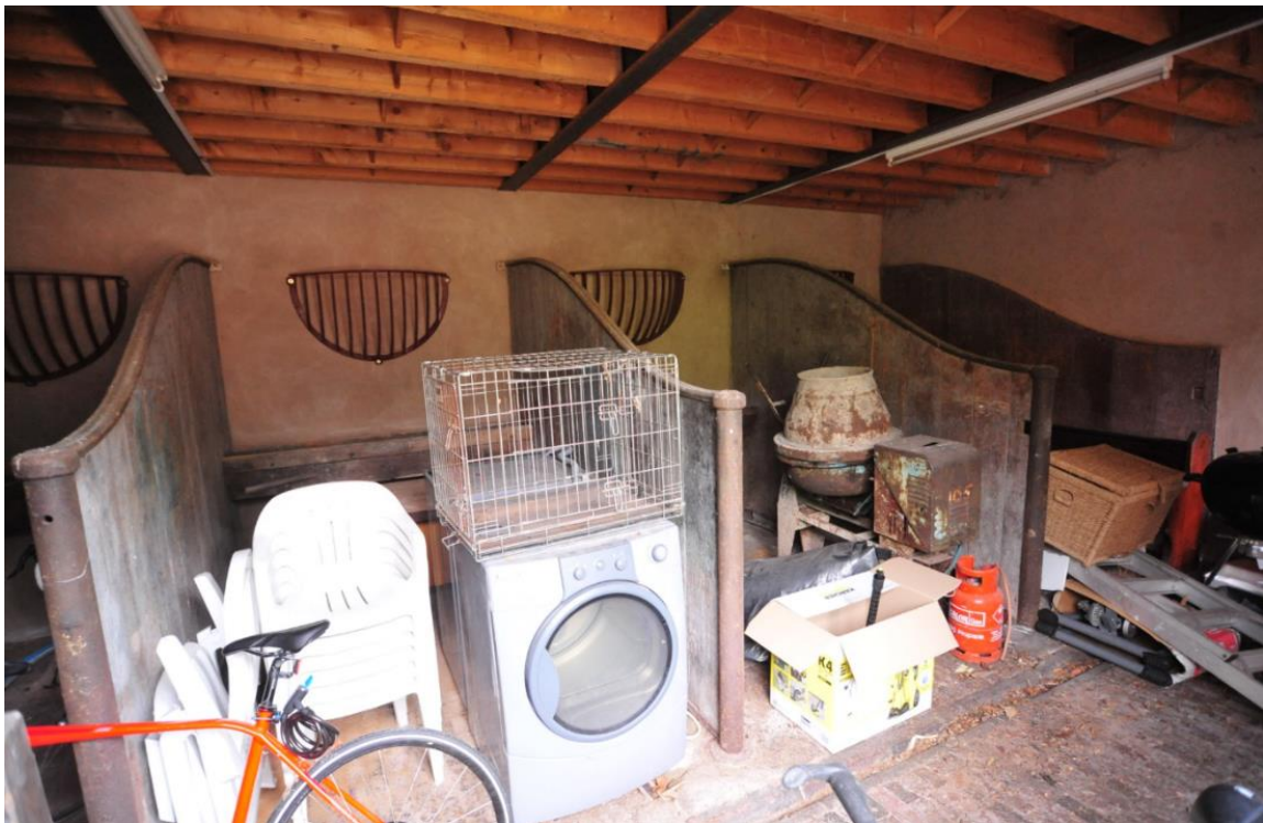
Pl.9: The stabling in the ground floor of the west wing.
