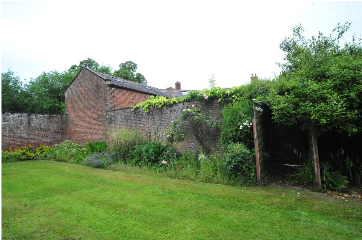
Pl.13: The south side of the south stable yard wall.
