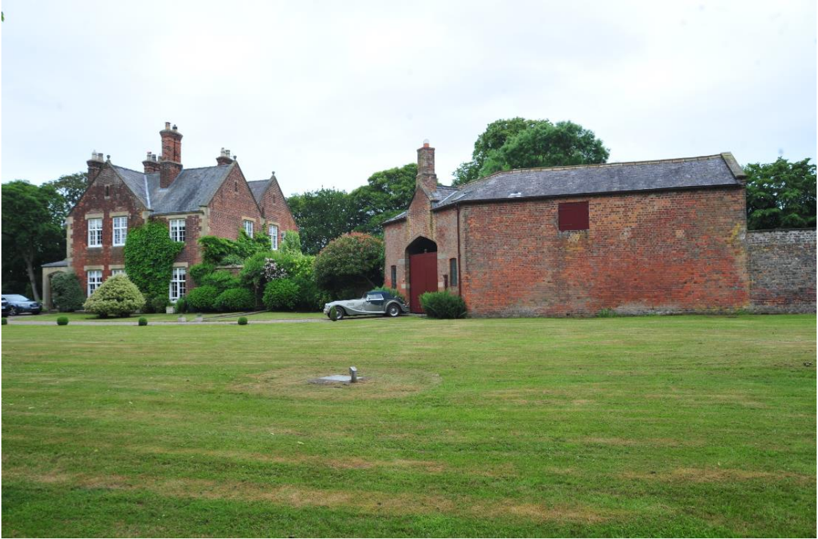
Pl.2: The Stables (right) from the west, with the rear of the house to the left.
