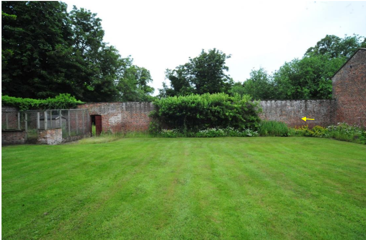
Pl.14: The eastern face of the western garden wall; note evidence for earlier structure built against this side of the wall in the past and the blocked former doorway (arrowed).
