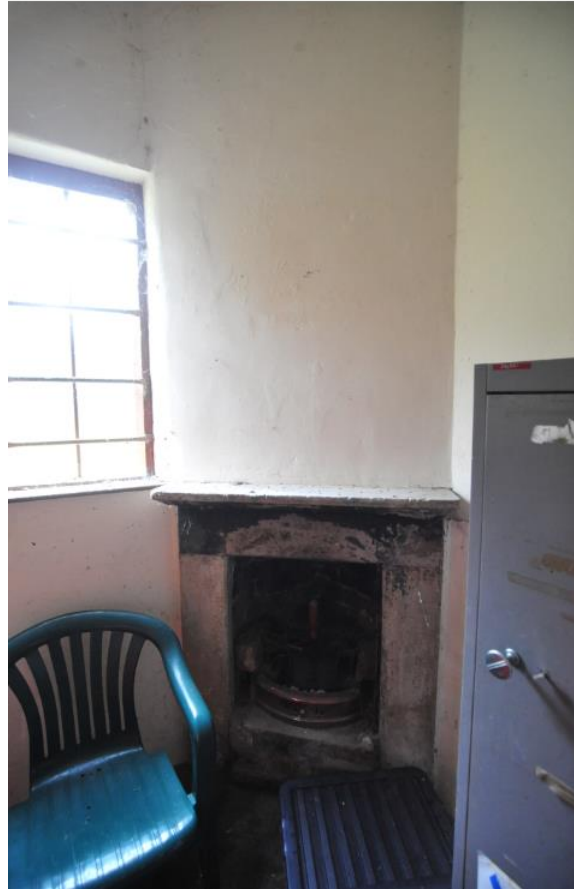
Pl.8: The groom's office fireplace.
