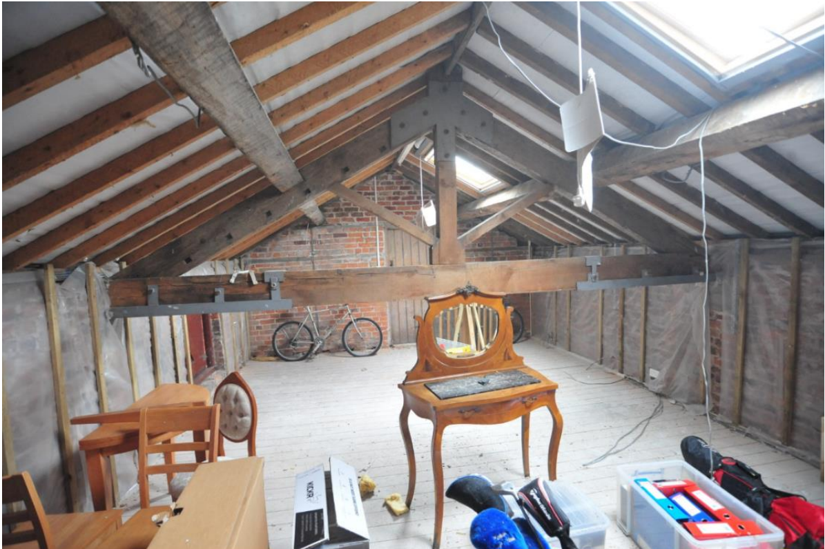
Pl.6: The roof over the west wing of the Stables.
