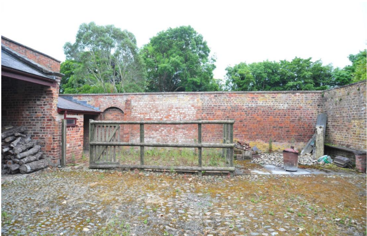
Pl.12: The inner face of the eastern stable yard wall.
