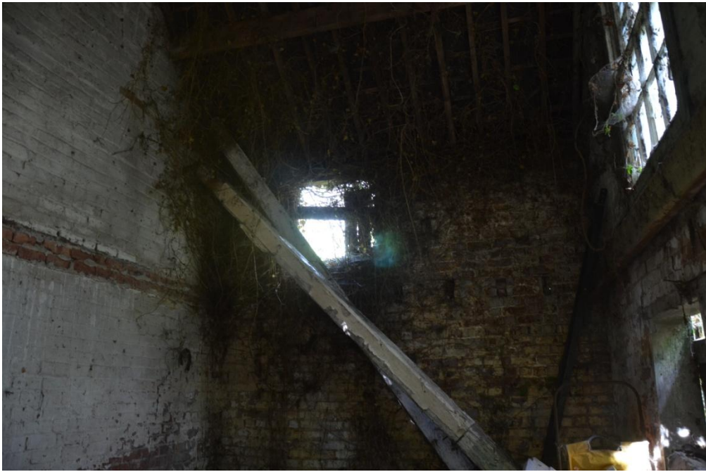
Photo 5 - Internal view of Area E. The majority of the bat activity / pre-emergence flight was observed in this area of the barn.
