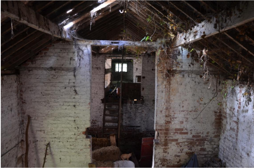
Photo 3 – Internal view looking across Area A – C.
