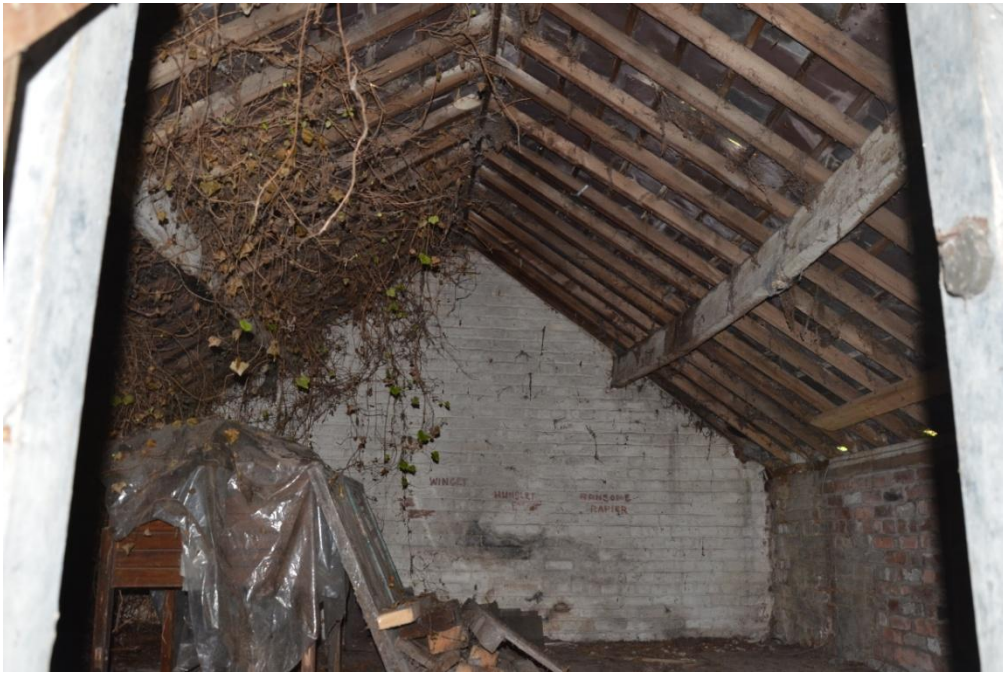
Photo 4 - Internal view of Area D. This room was notably darker earlier than other areas of the barn lacking external windows and doors.
