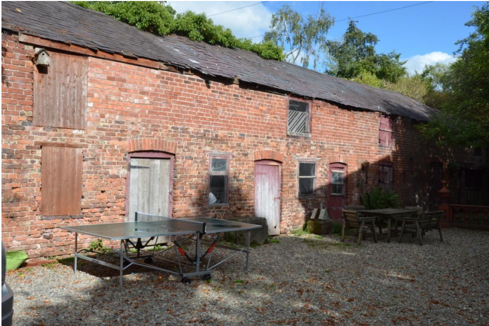
Photo 1 - Front elevation of Higher Oak Barn.
