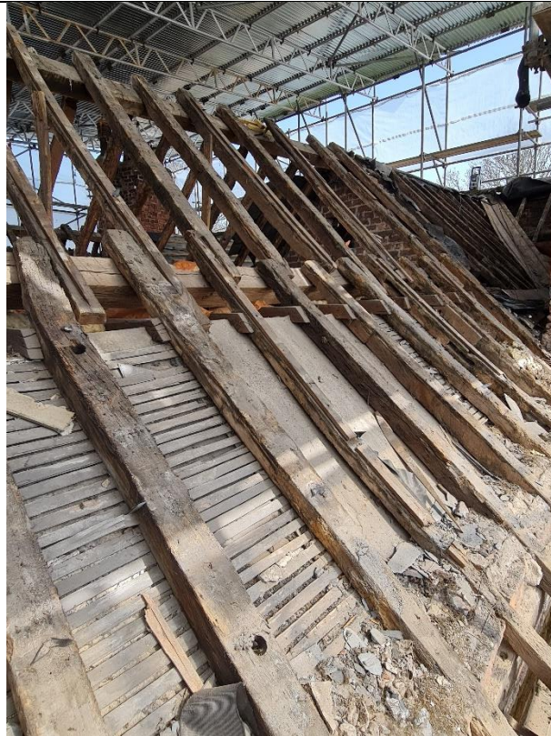
Roof View to front
