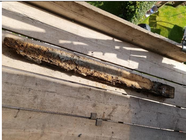
Rotten timber removed
