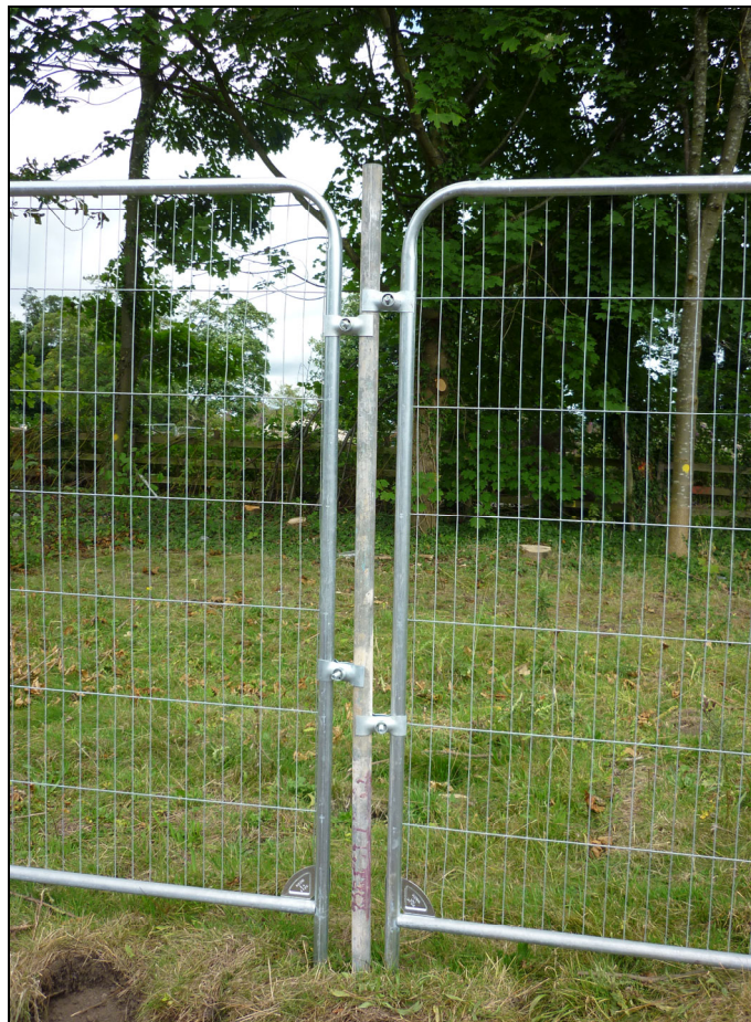
Tree Protective Fencing Specification
