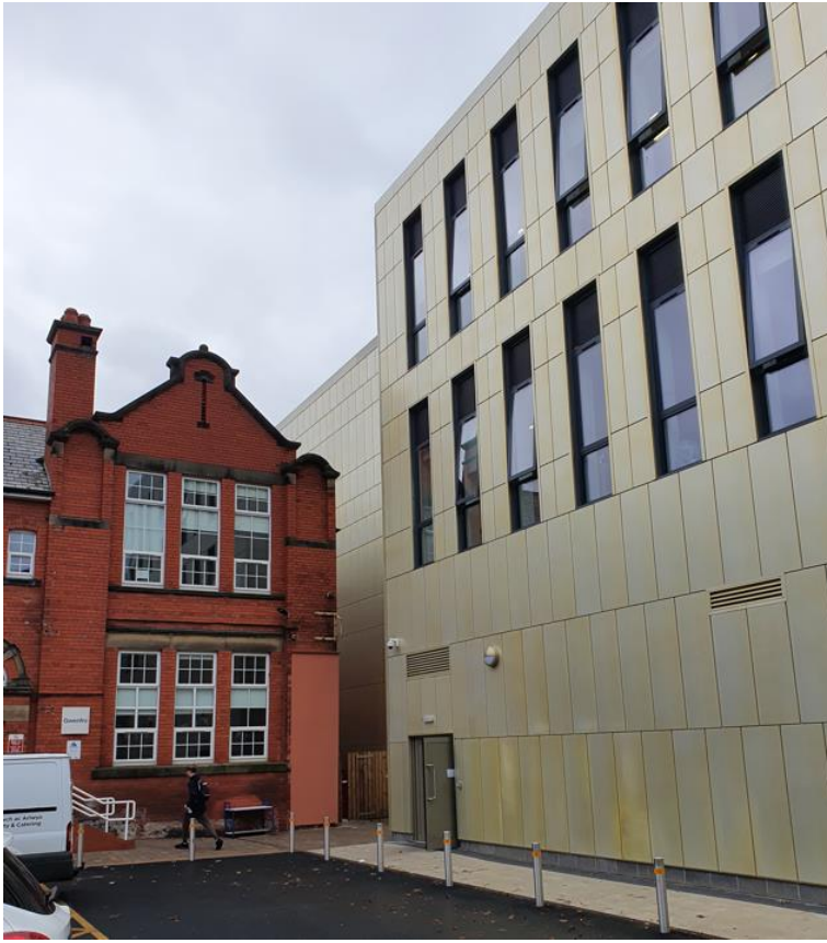
Example of newly completed existing metal clad building with tall slot windows to the right side of the Victorian building.
