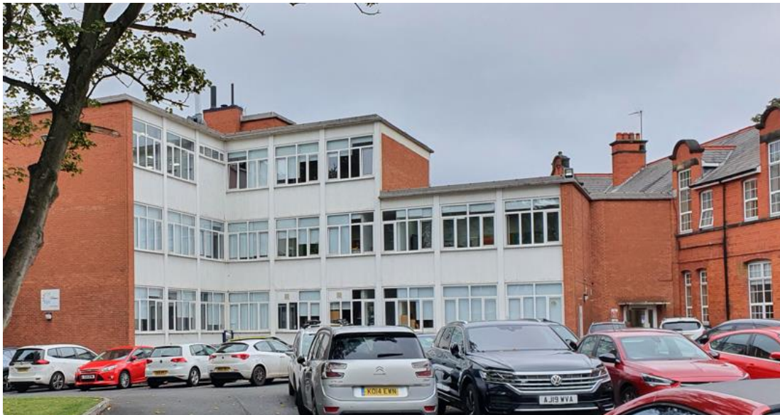
View towards the three-storey building which is to be demolished and the retained Victorian building to the right. When complete, the proposals will follow designs the newly completed building to the right of this Victorian building.
