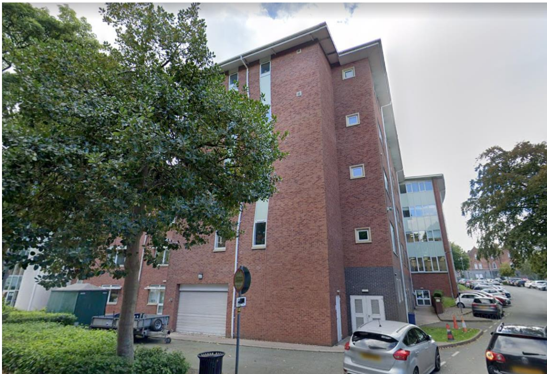
Existing five storey building opposite the proposed development that is within the Grosvenor Conservation Area
