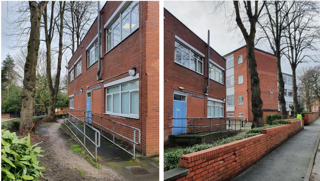
Gable elevations of buildings fronting the Grosvenor Conservation Area curtilage. These are to be demolished. Wall to be rebuilt in same bonding following completion with a new stone capping in keeping with original design
