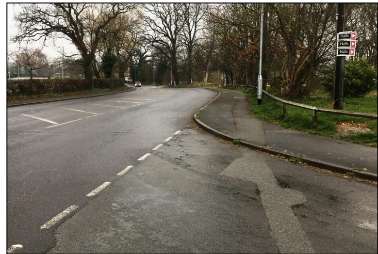
Junction visibility to the right
