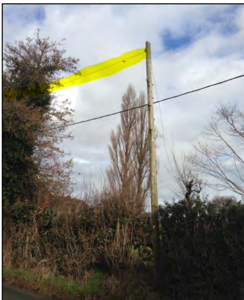
Fig. 8.05 – BT infrastructure and pole requiring removing
