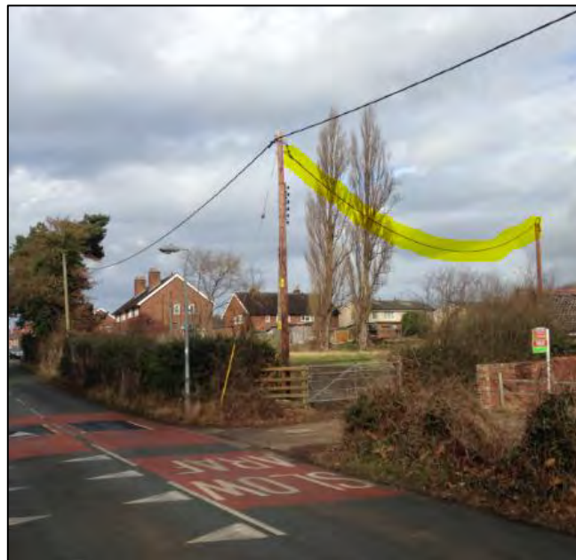
Fig. 5.08 – Location of overhead LV supply requiring disconnection
