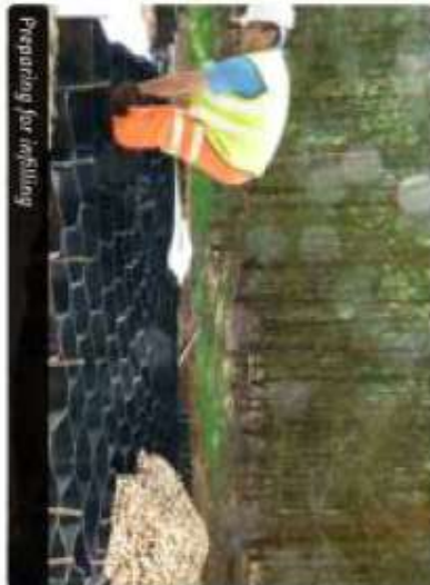
Inserting temporary pins to hold cell panel open
