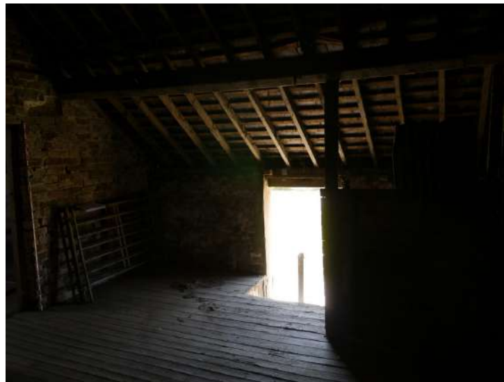
Plate 39 - Threshold south-west elevation room F3
