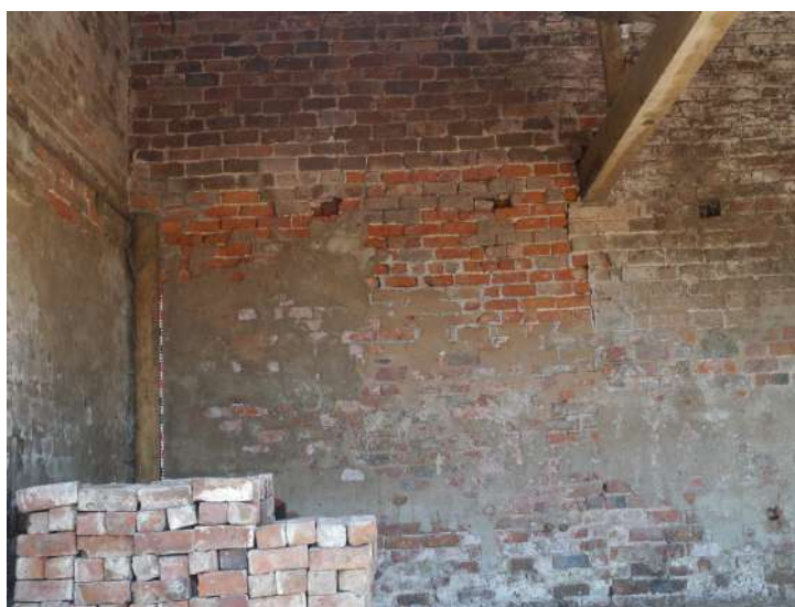
Plate 22 - South-west reconstruction wall room B4
