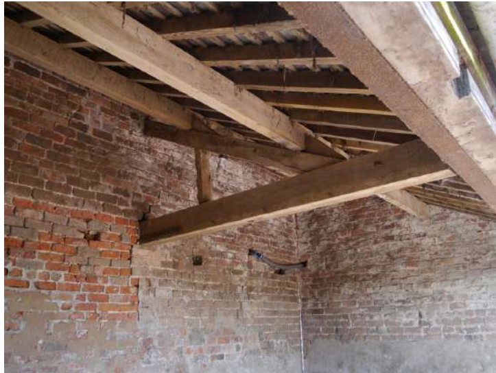
Plate 21 - Open roof with steel joist room B4
