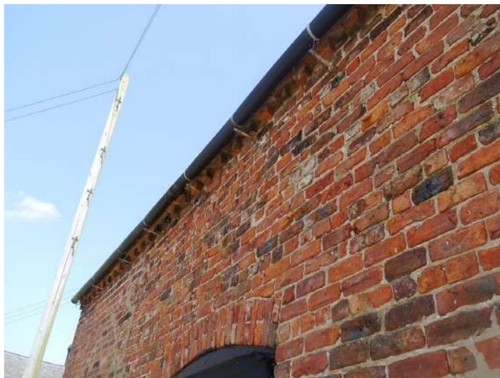
Plate 4 - Dentil top course south- west elevation
