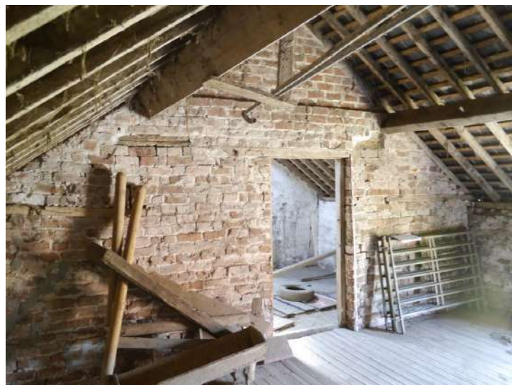
Plate 40 - South-east elevation room F3
