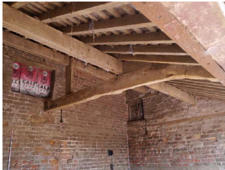
Plate 15 - Air ventilation window north-west wall room B1
