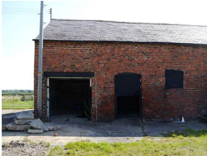
Plate 5 - Room B5 threshold
