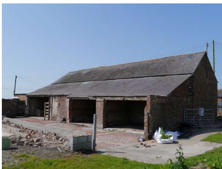
Plate 2 - North-east elevation of rooftop
