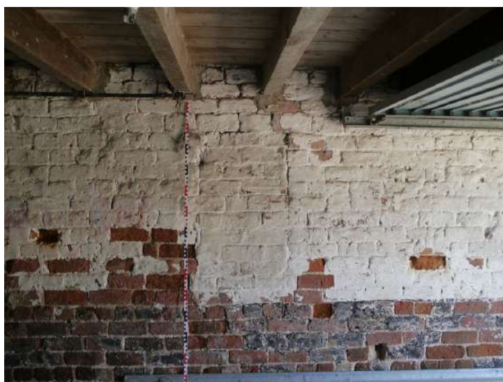
Plate 24 - Sealed air ventilation feature north-west elevation room B5
