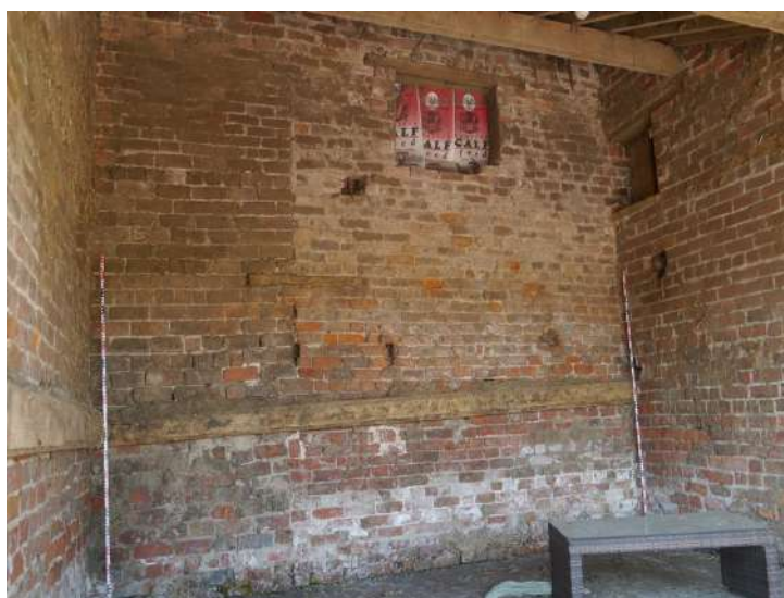
Plate 17 - South-west reconstruction wall room B2
