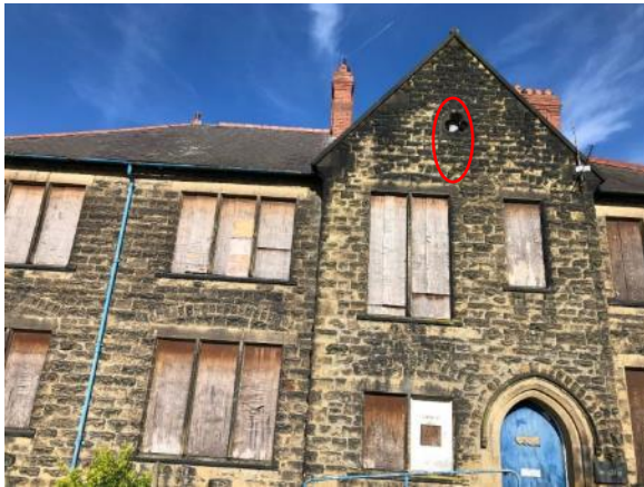
Plate 1: South-east elevation of Centre 67 showing loft window
