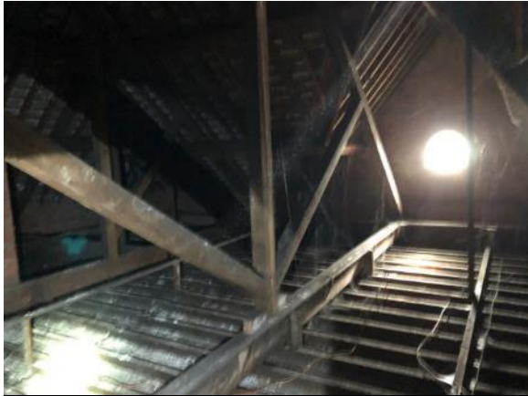
Plate 4: Condition of the loft space showing the window
