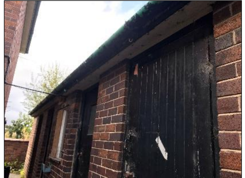
Eastern elevation of B2 (pictured above).
