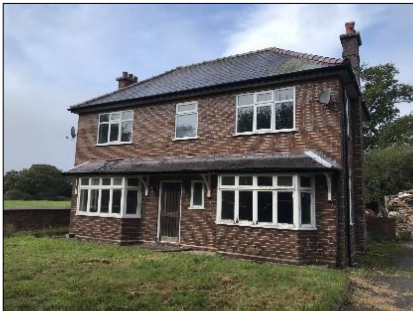
Eastern elevation of B1 (pictured above).
