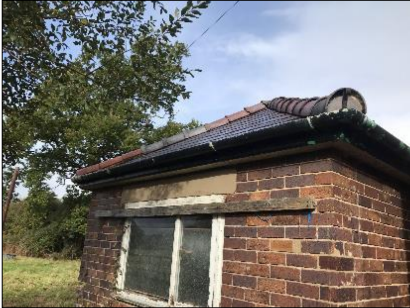
Southern elevation of B2 (pictured above).
