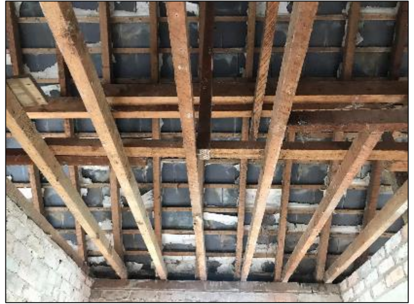
Interior of B1 (pictured above).
