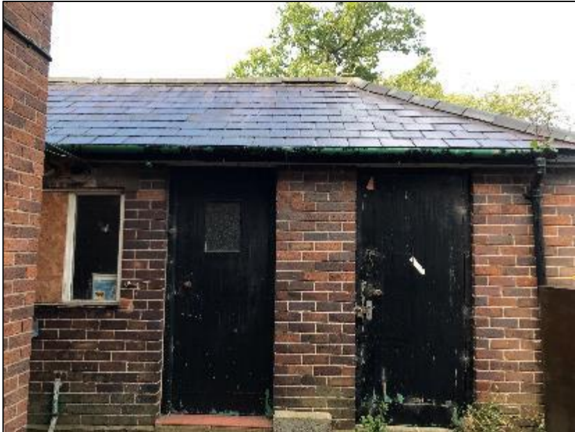
Eastern elevation of B2 (pictured above).
