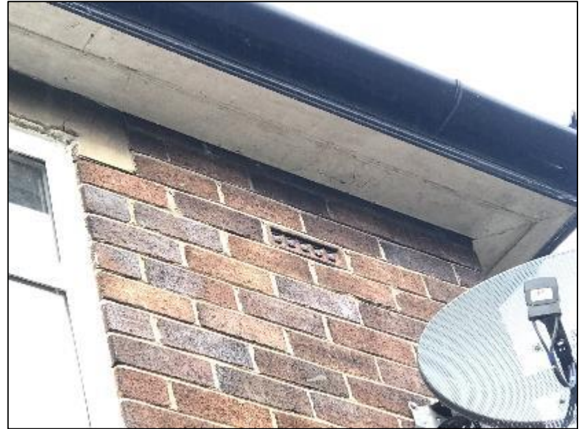
Close-up of building eaves on eastern elevation of B1 (pictured above).
