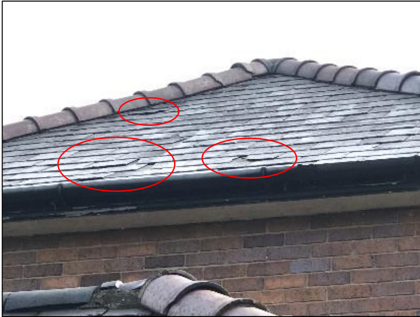
Close-up of roof structure on western elevation of B1 (pictured above).
