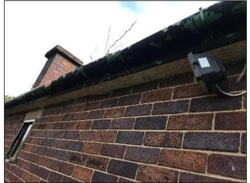
Close-up of eaves on western elevation of B2 (pictured above).
