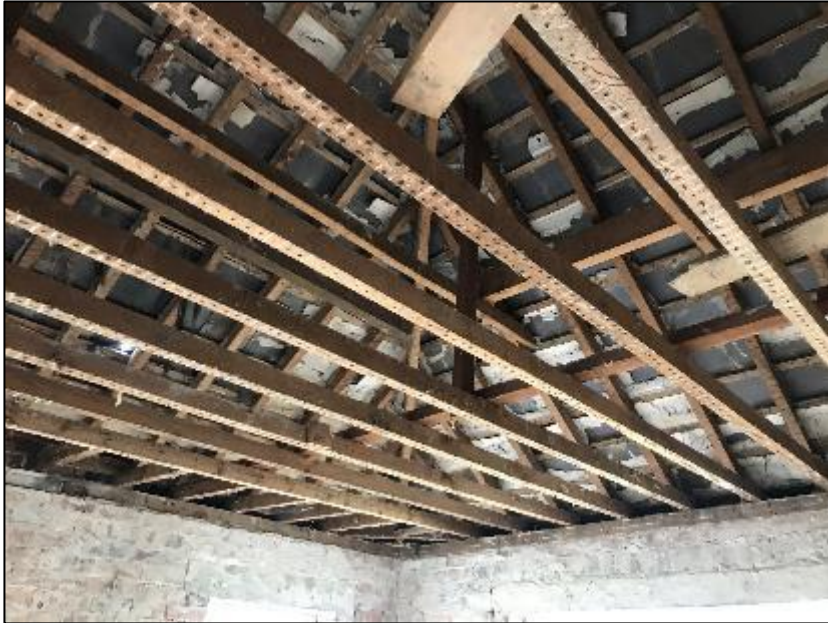
Interior of B1 (pictured above).
