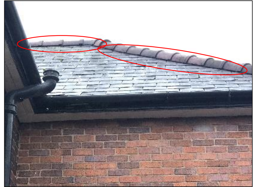
Close-up of roof structure on northern elevation of B1 (pictured above).
