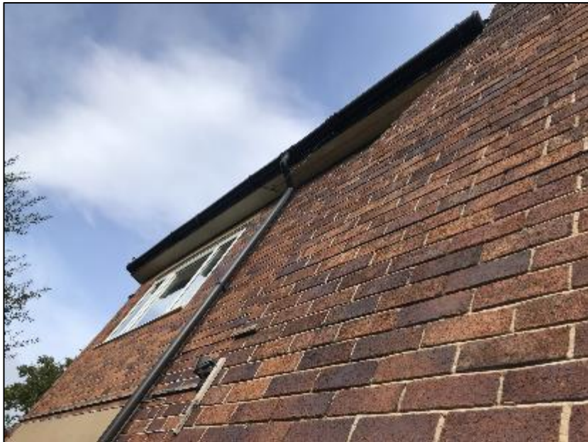
Southern elevation of B1 (pictured above).
