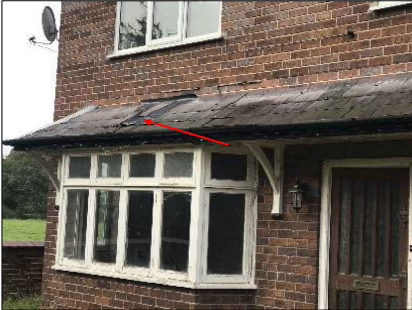
Single-storey sub-roof on eastern elevation of B1 (pictured above).
