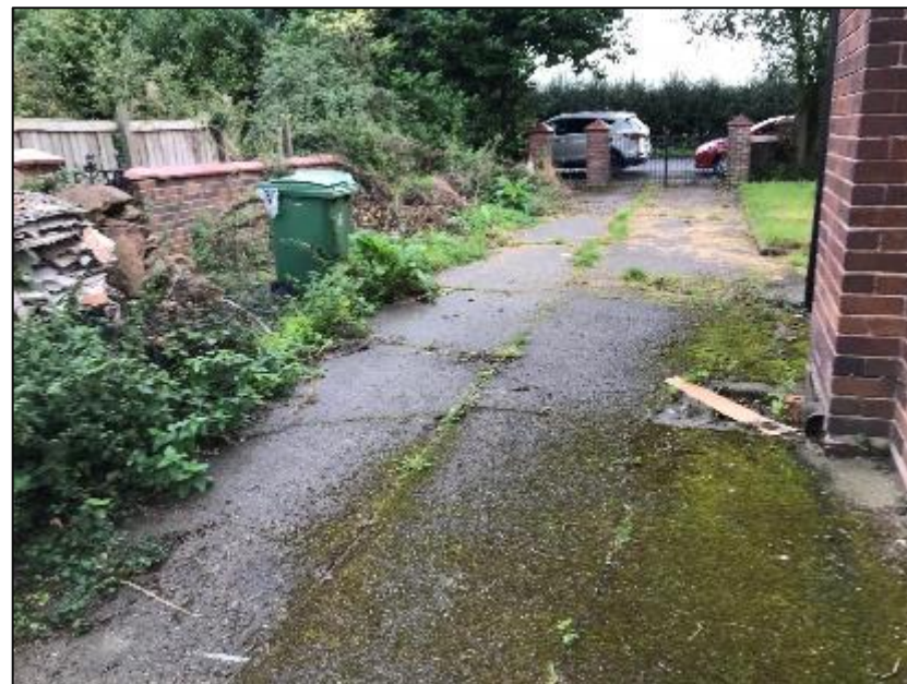
Hard standing driveway (pictured above).
