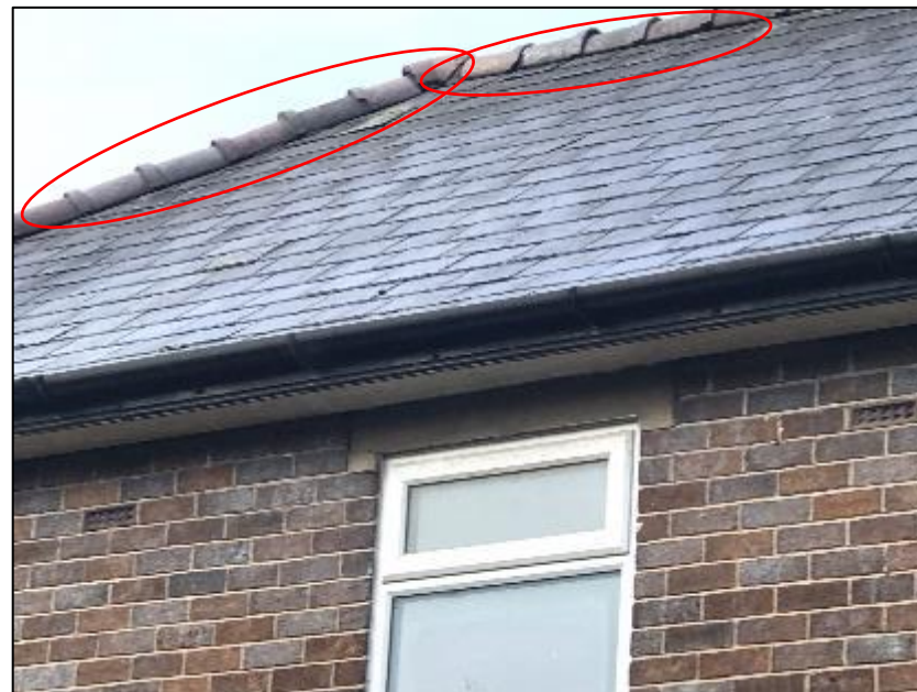
Close-up of roof structure on eastern elevation of B1 (pictured above).
