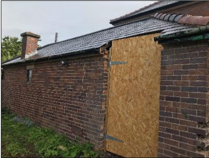
Western elevation of B2 (pictured above).
