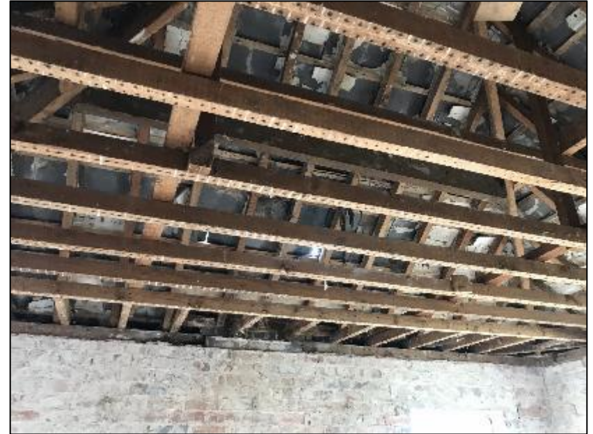
Interior of B1 (pictured above).
