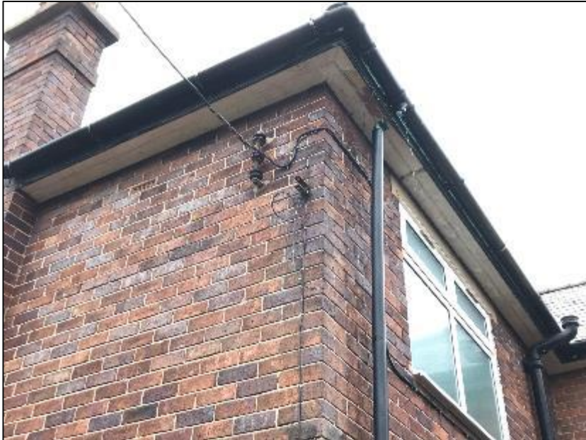
Close-up of eaves on northern elevation of B1 (pictured above).
