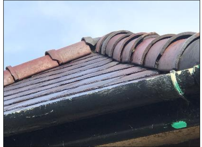
Close-up of roof structure on southern elevation of B2 (pictured above).
