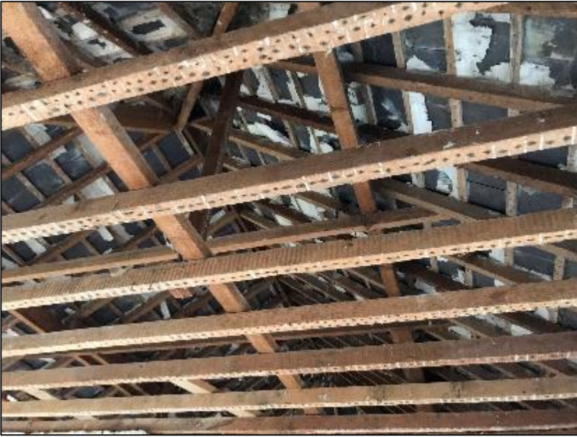
Interior of B1 (pictured above).
