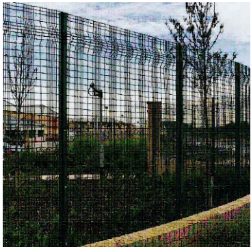
Typical example of proposed fence. Paladin style open mesh or similar Colour RAL9005 Jet Black
