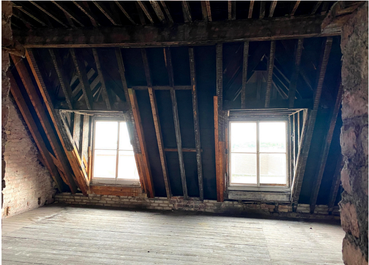
Vacant top floor - stripped back to brickwork
