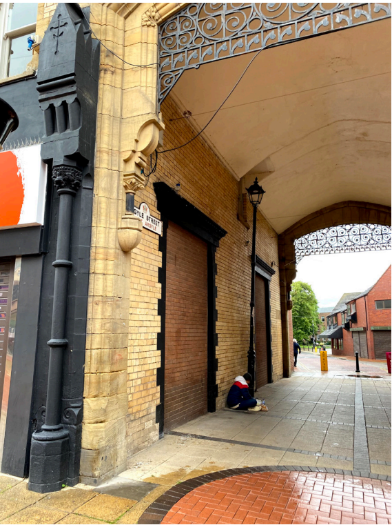
Archway looking towards Argyle Street
