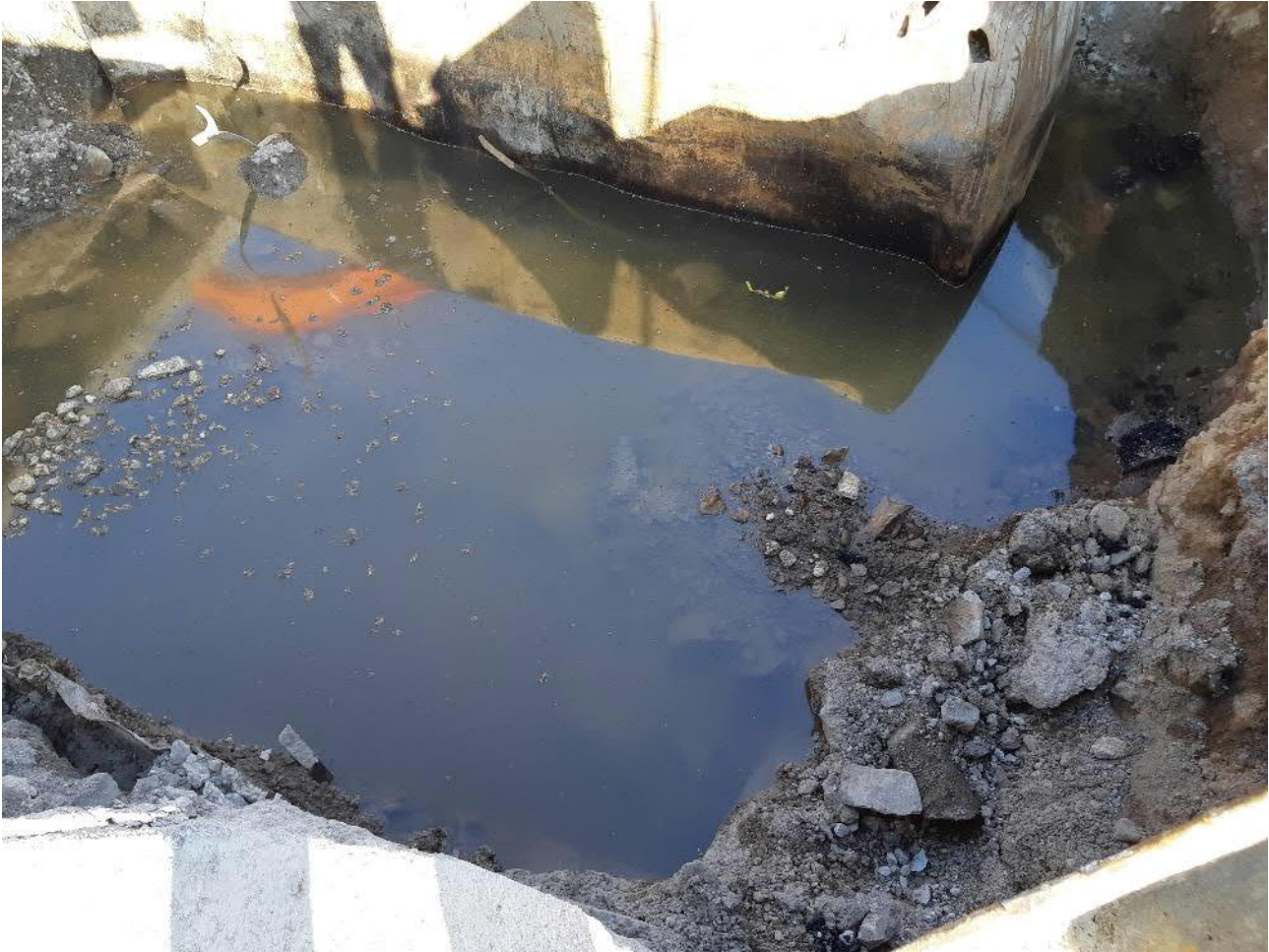
Figure Error! No text of specified style in document..3: Groundwater with Excavation
