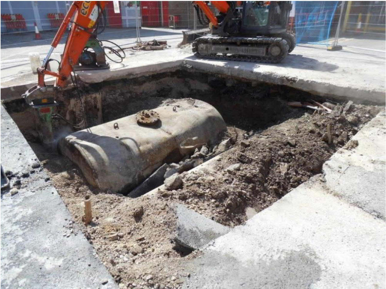
Figure Error! No text of specified style in document..1: Tank Removal
