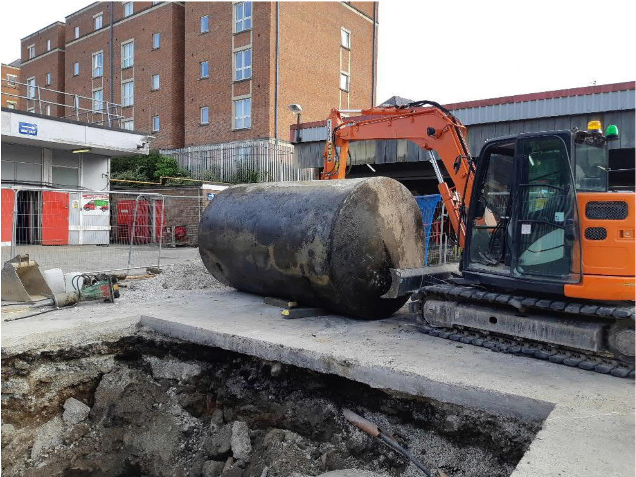
Figure Error! No text of specified style in document..2: Removal of First Tank
