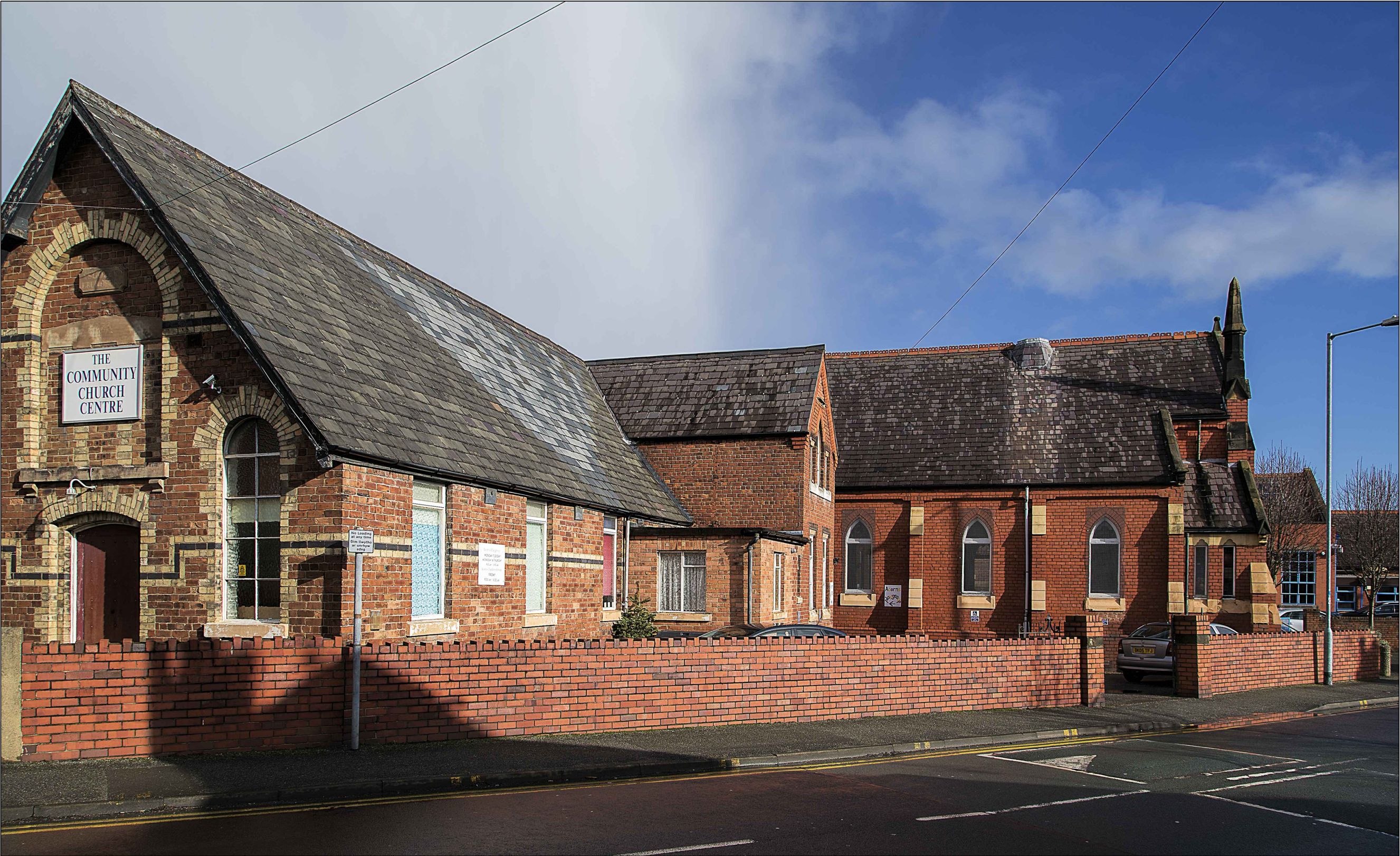
01. Photograph of Existing (South West)
