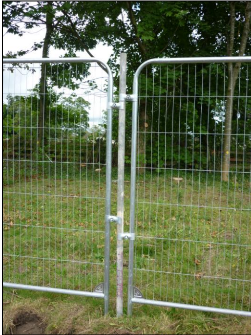
Tree Protective Fencing Specification
