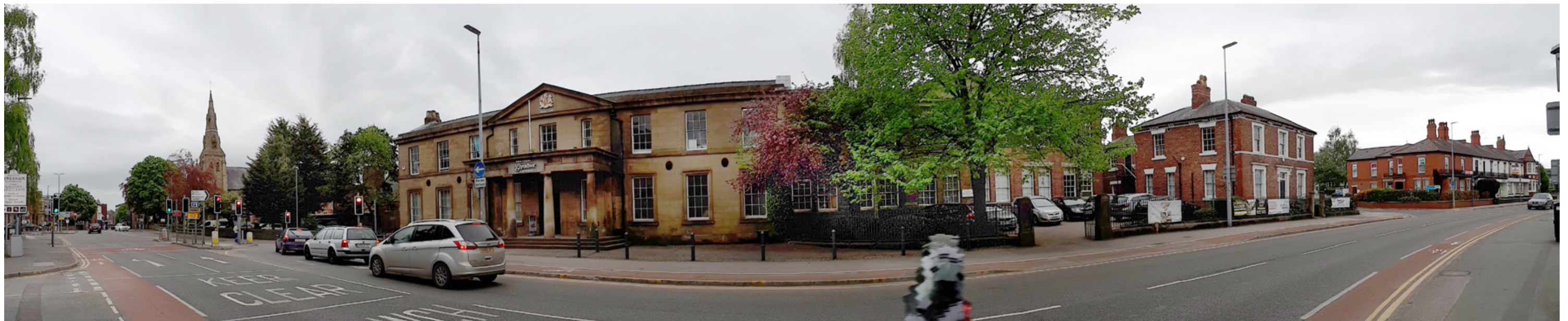
5. View of the Listed Building frontage from Regent Street
