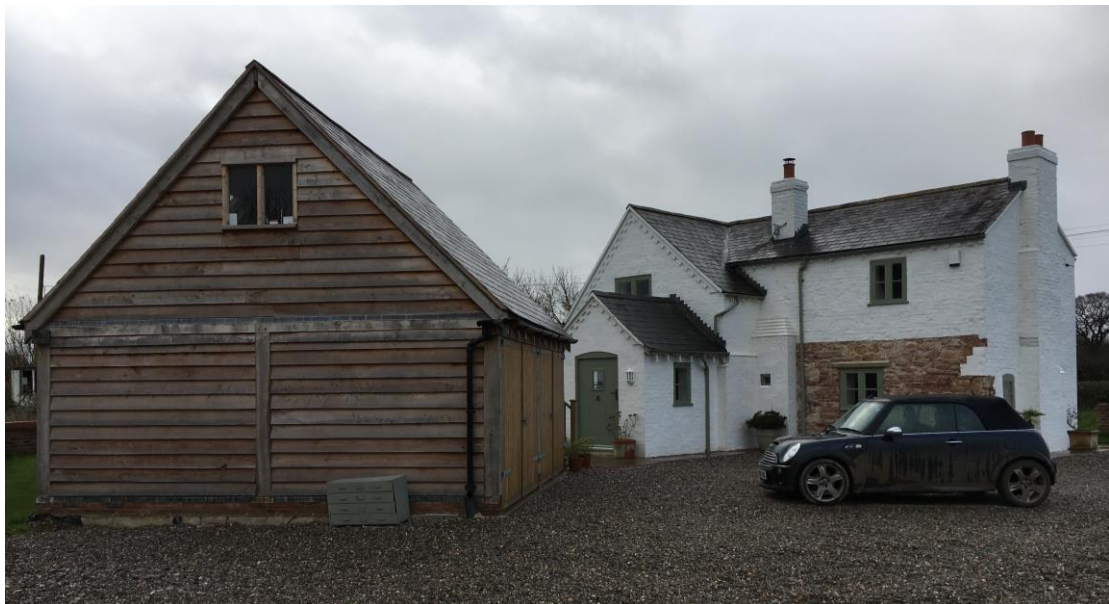
Recent Views of the Site, Illustrating the Extent of the Works Undertaken to the Buildings
