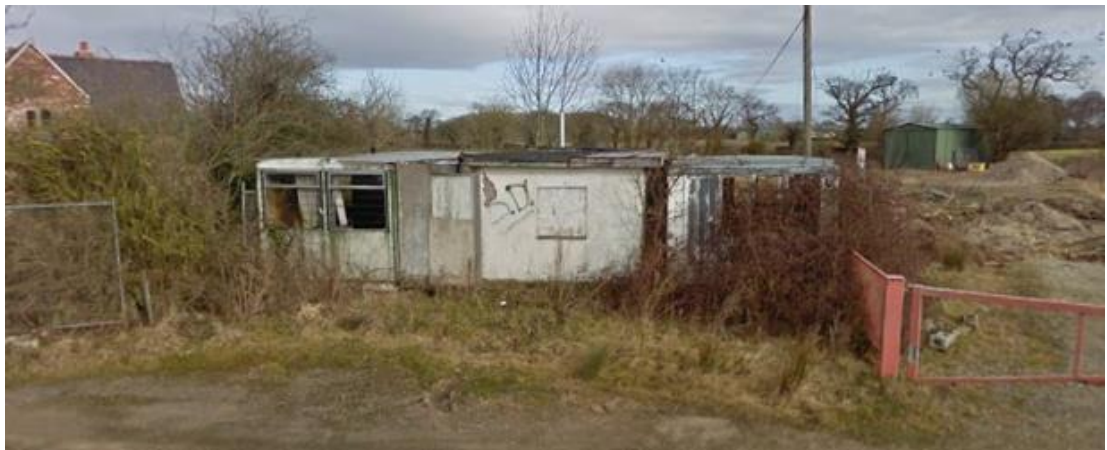
Historic Views of the Site, Illustrating the Extent of Dilapidation of the Grade II Listed Building
