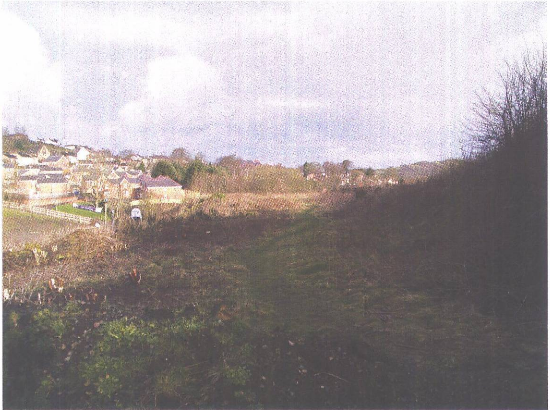
Top of railway embankment looking north
