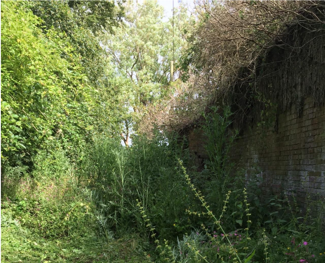
Fig. 2.5 Photograph of land to the north of the outbuilding
