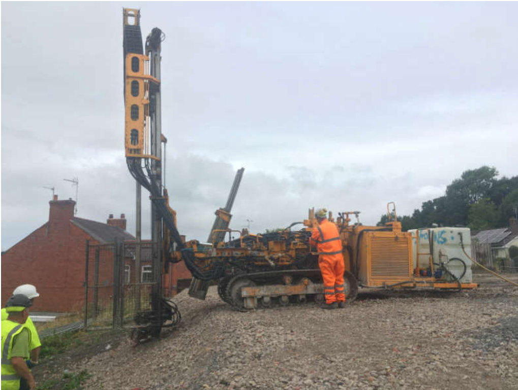
Photograph 1 Klemm Drilling rig
