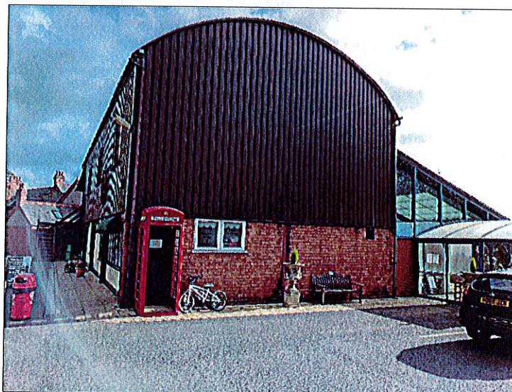
Photo 5: Building B1 western elevation
