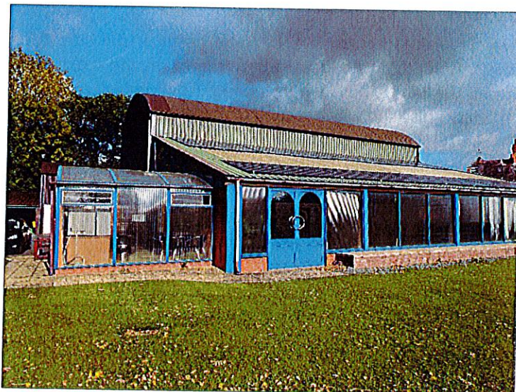
Photo 6: Building B1 southern elevation
