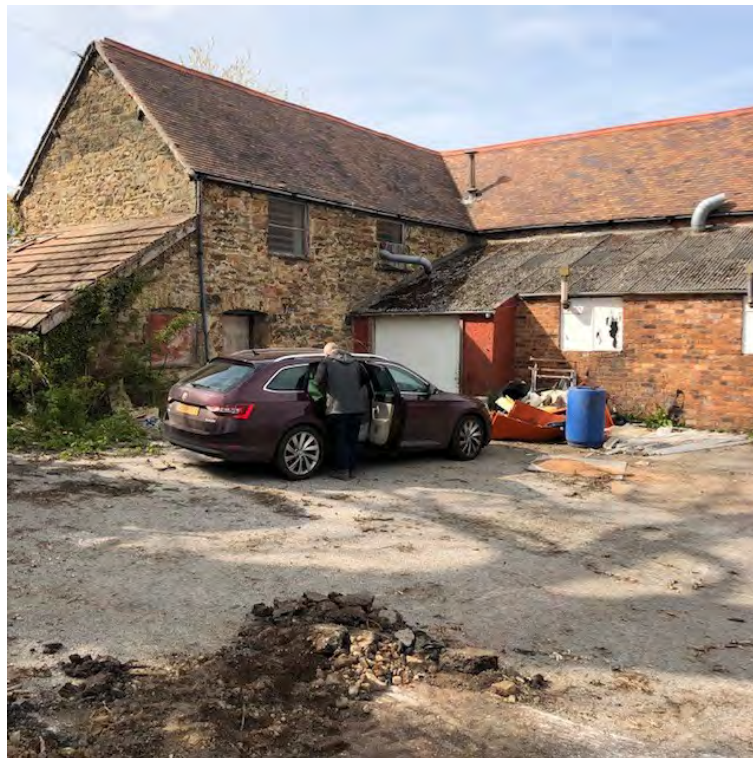
Photograph 3- Facing west showing existing masonry building.
