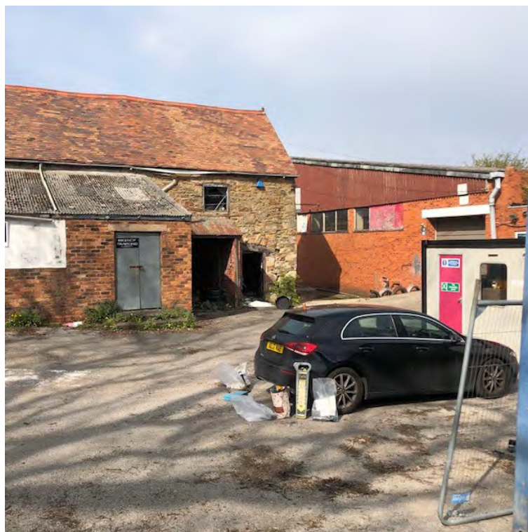
Photograph 4- Facing north showing existing masonry building and adjacent industrial unit.
