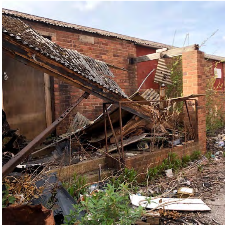
Photograph 10- Facing west showing partly demolished extension to the masonry building.
