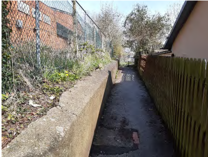
Photograph 9- Showing Retaining wall on eastern site boundary.
