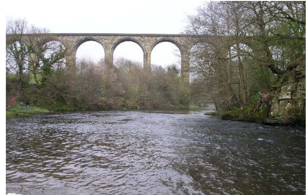
Railway Viaduct over River Dee
