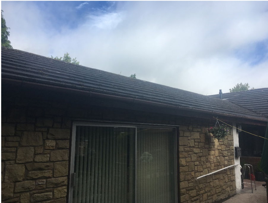
Plate 3: Eastern elevation of building and single storey veranda
