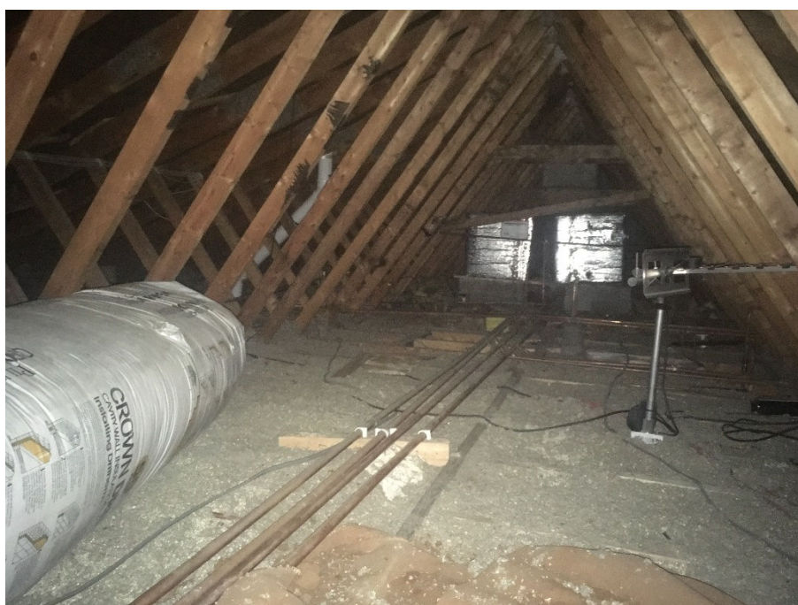
Plate 6: Roof void of building
