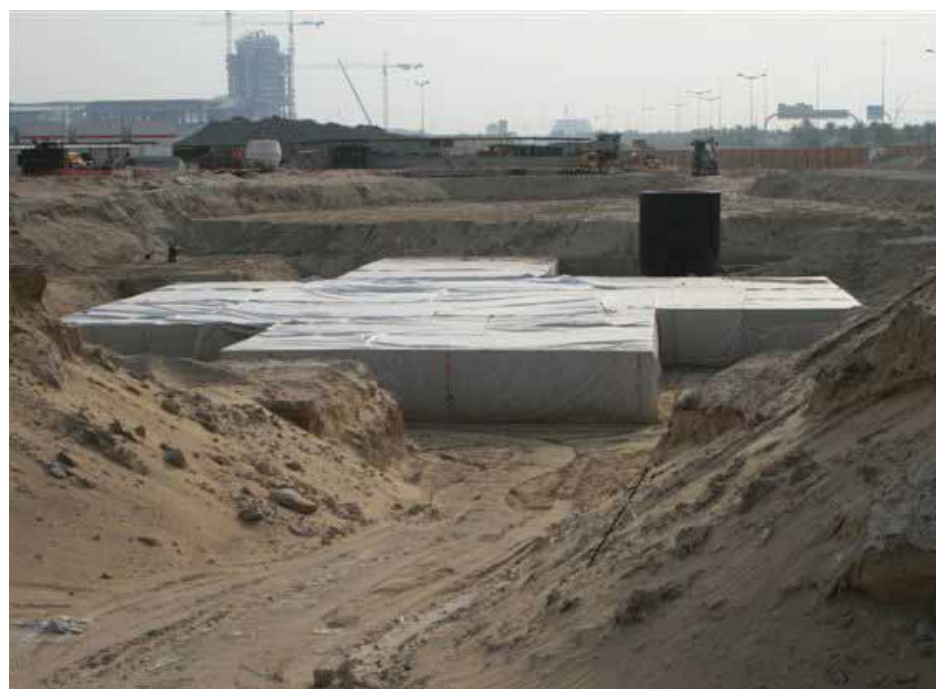
1600m 3 Soakaway 2 meters deep, 3 meters of cover
