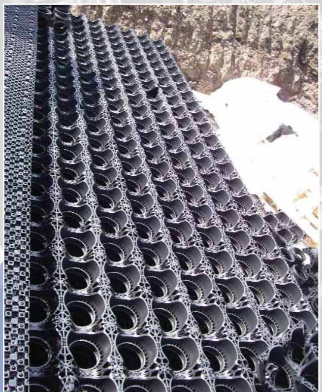
Horizontal access channel through system
