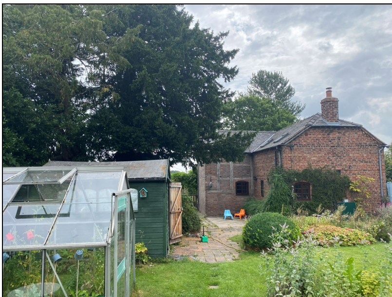
P3 – Site viewed from garden area to west
