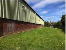
Rear of building where forklift truck route to run
