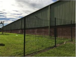
Existing fencing to be relocated and / or replaced to match existing
