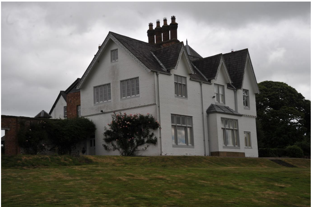
Pl.8: The house from the south-west.
