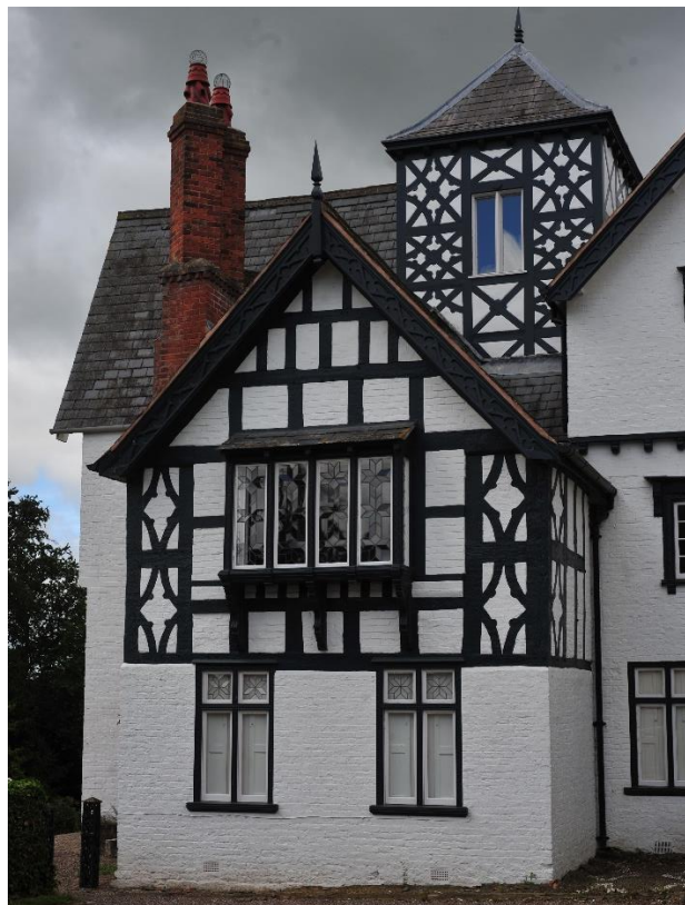
Pl.16: Detail of much altered original south-east wing and 19 th century turret beyond.
