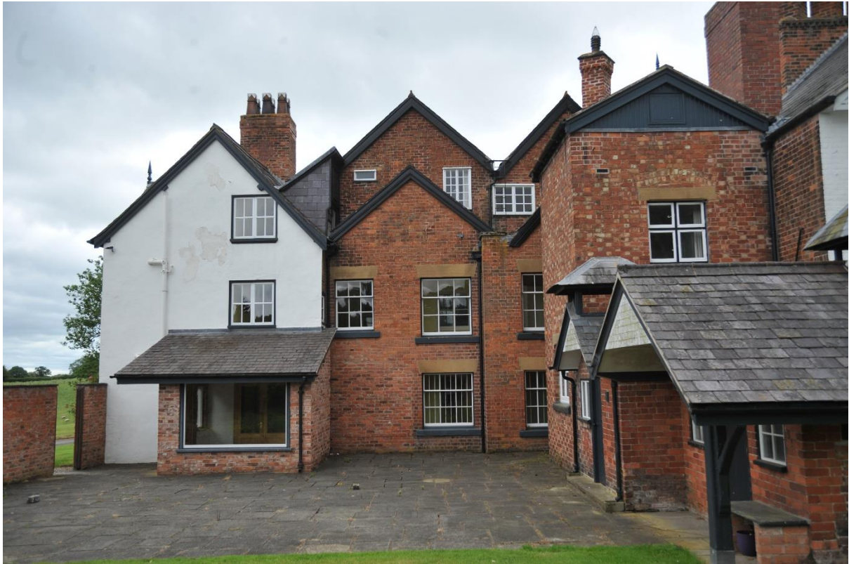
Pl.11: Detail of the northern end of the west elevation.
