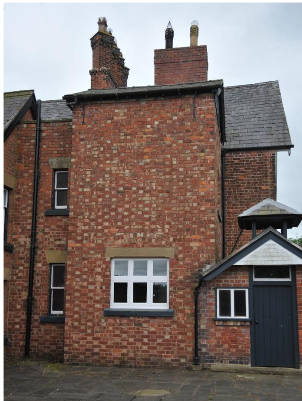
Pl.12: The north elevation of the projecting western wing of the house.
