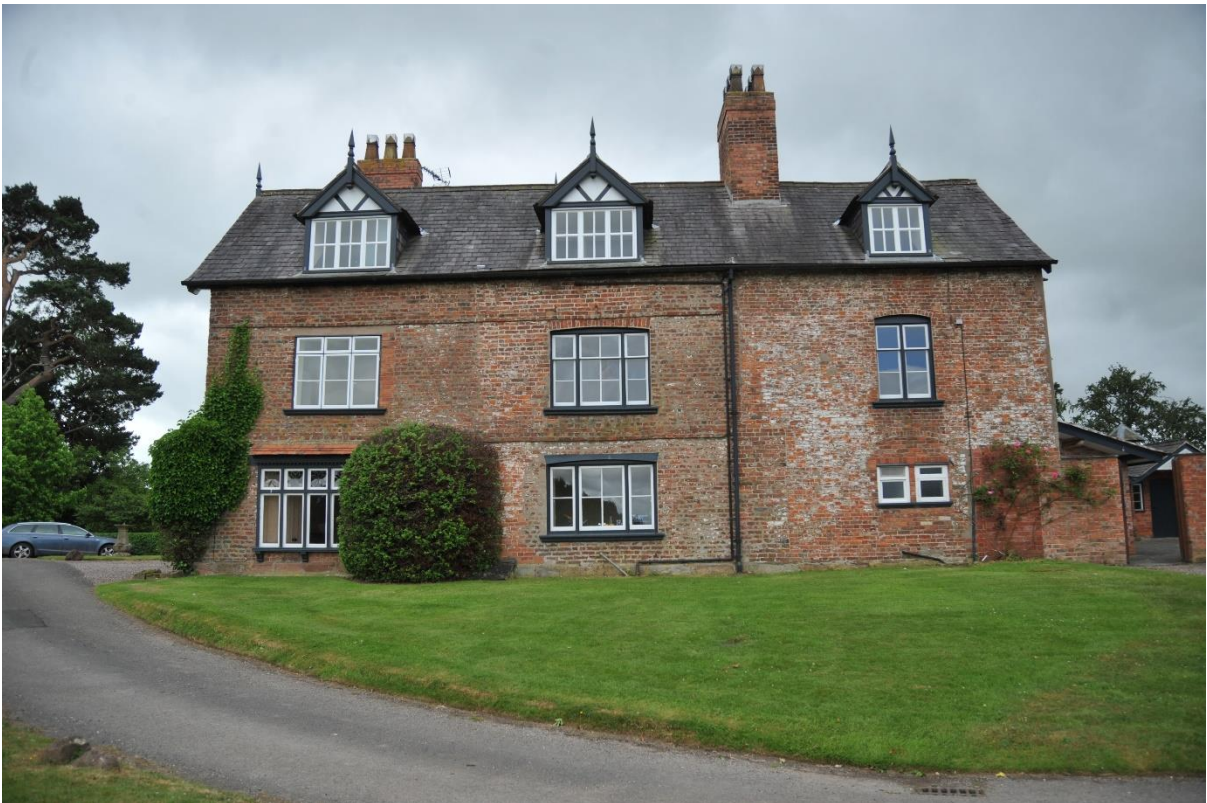
Pl.14: The north elevation of the house.
