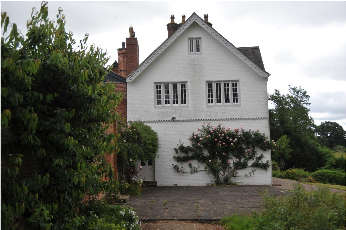
Pl.10: Detail of the southern end of the west elevation.
