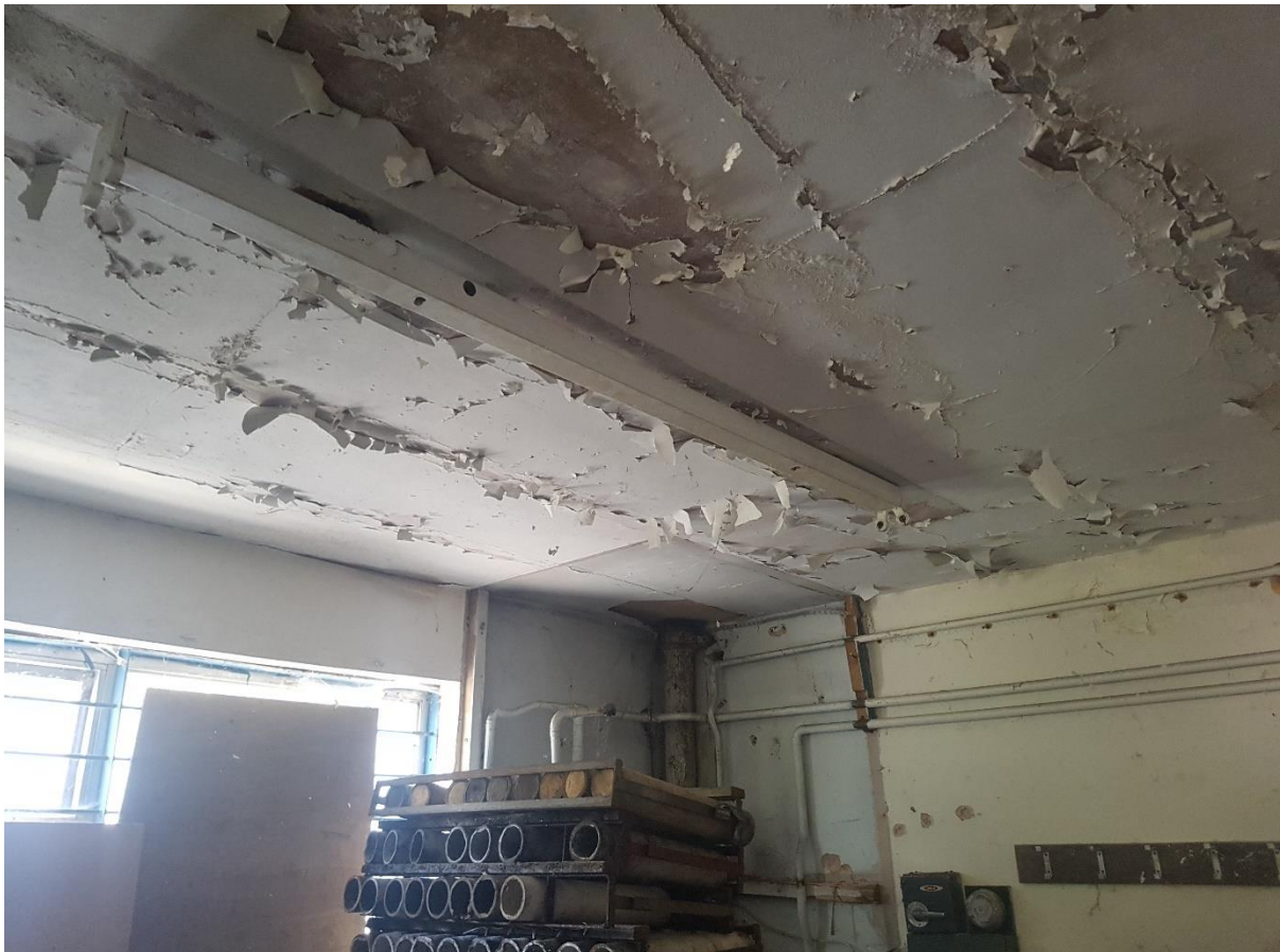
Image 3.6 The northernmost portion of B1 constructed of concrete
