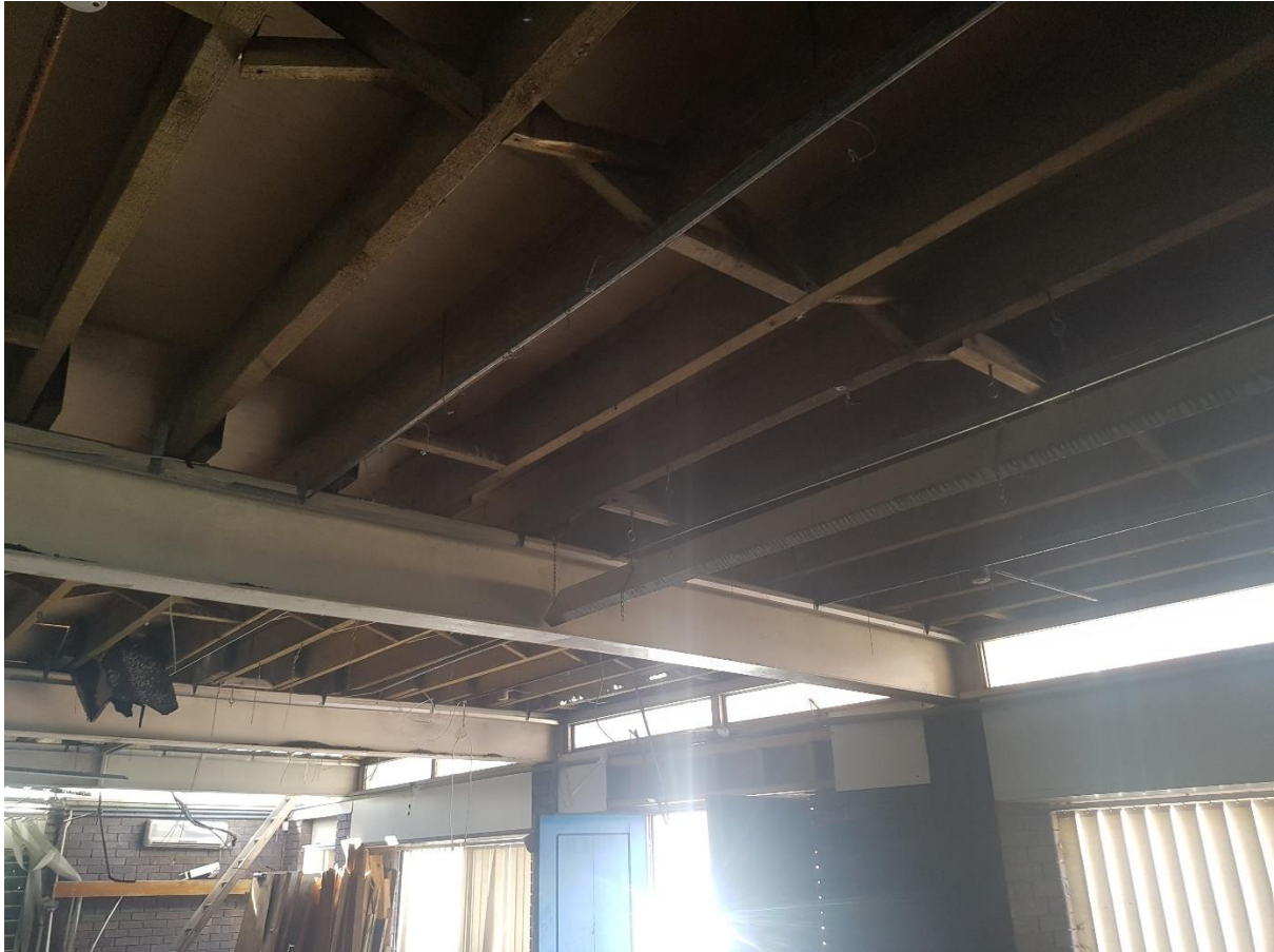
Image 3.5 The southernmost portion of the roof boarded with timber
