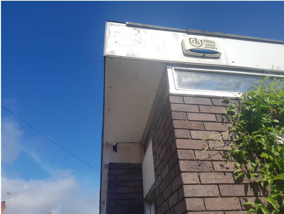
Image 3.4 The soffits and eaves of B1 in good condition
