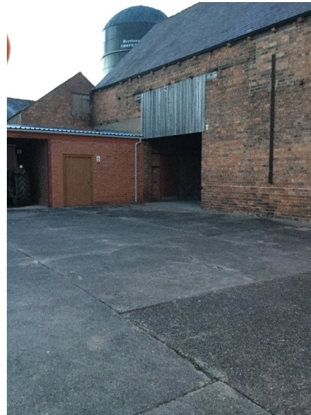
Plate 3: Building 14 showing open void
