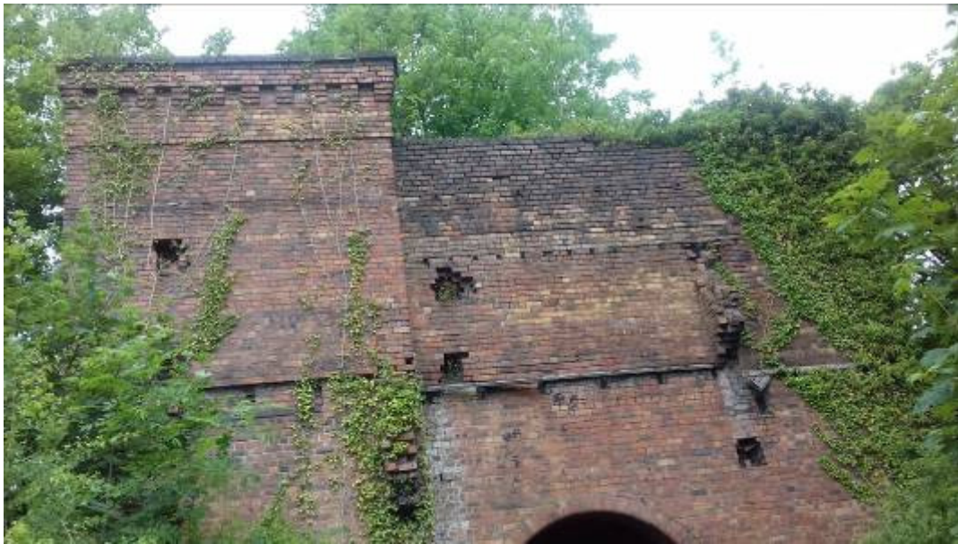
Walker Fan House building (B5) – potential to south, east and western aspects in the form of brick work crevices & hibernation potential
