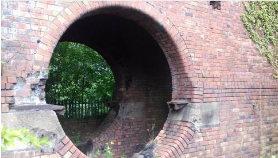
Interior of B5 – could not be accessed due to safety reasons
