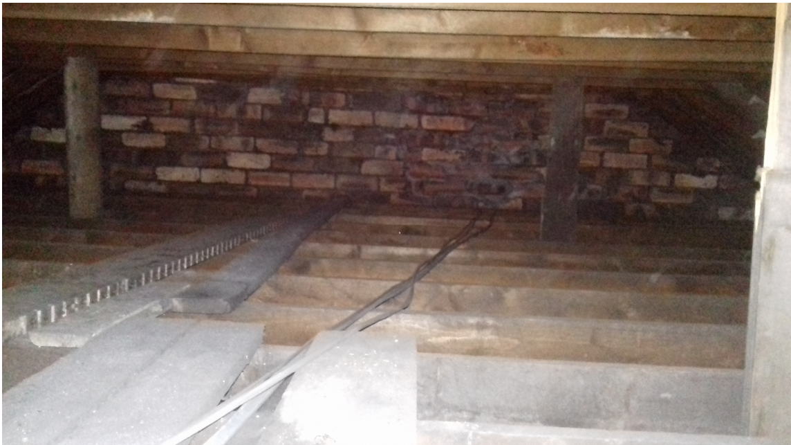
Truss roof construct of B1
