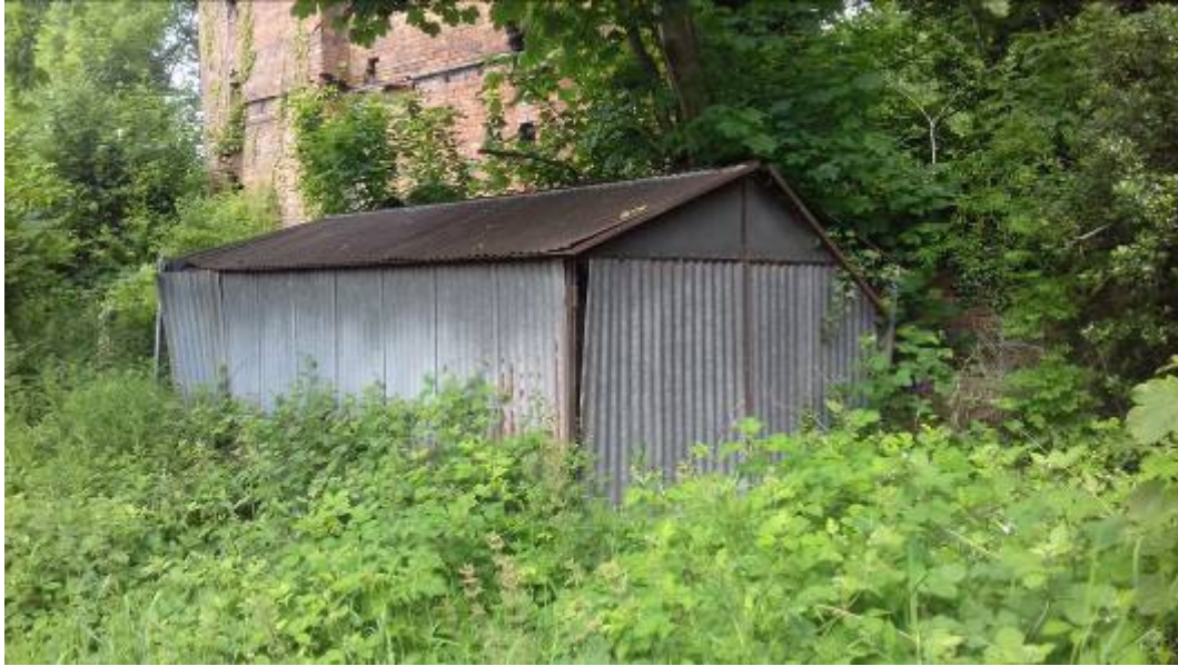
Corrugated metal shed (B4) – no roost potential
