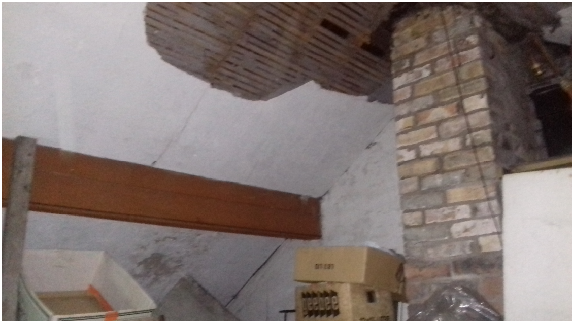
Lime and mortar finish beneath roof slates of B1
