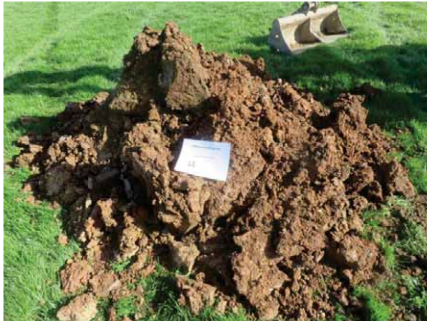
Photo 84 – Arising's Trial Pit 41
