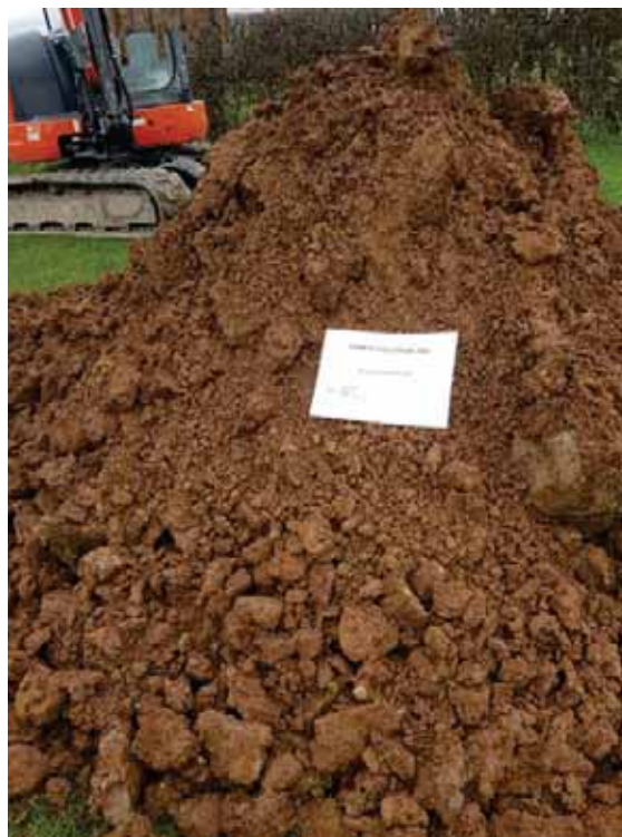
Photo 4 – Arising's Trial Pit 02
