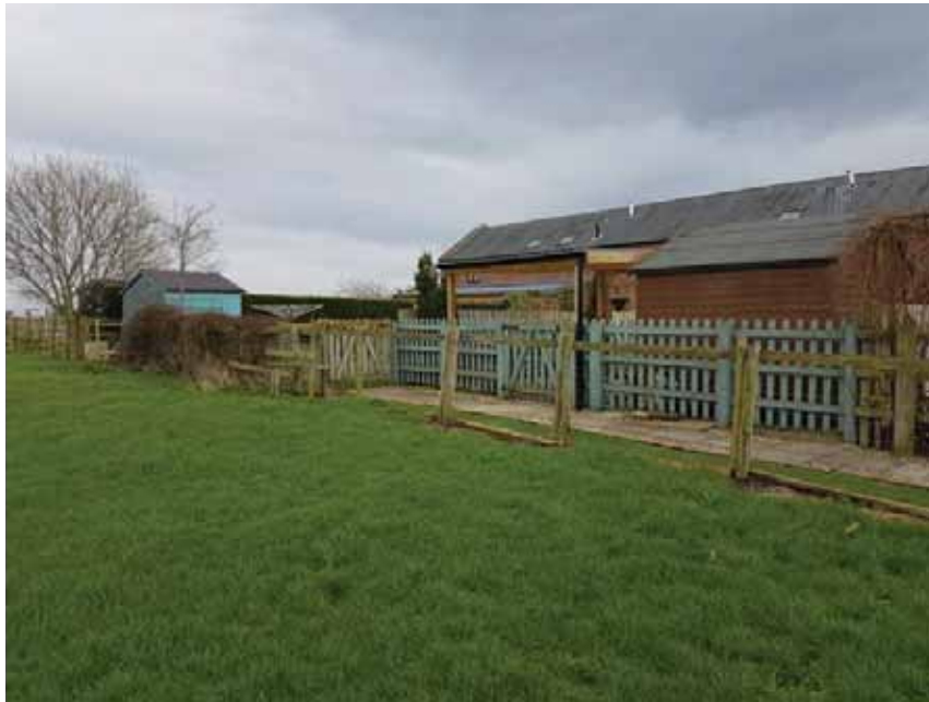
Photo 9 – View of barn conversions which back onto area 2 from the east
