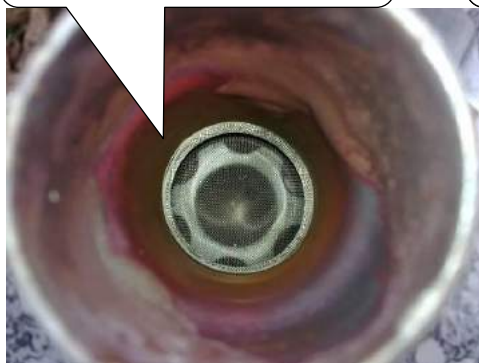
A clean filter (on the suction pipe of the system)
