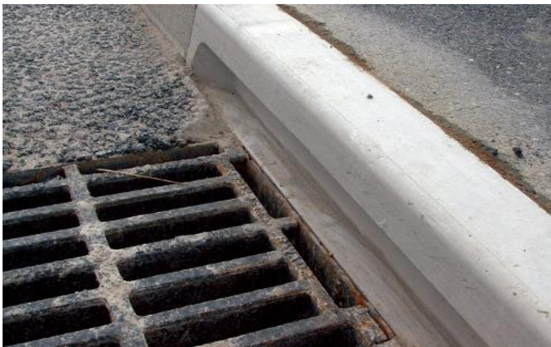
Figure 4: Example bypass kerb.
