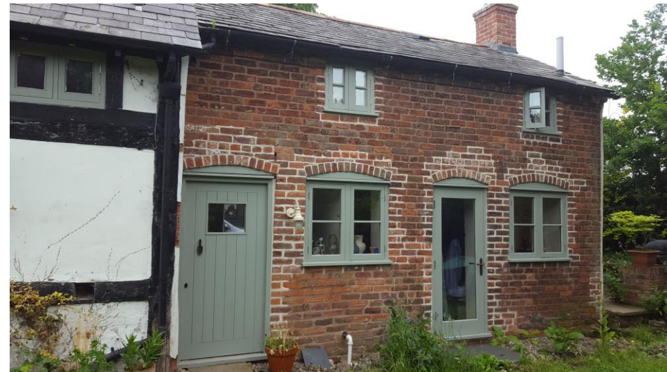
Figure 6 – View looking East towards previously built rear extension
