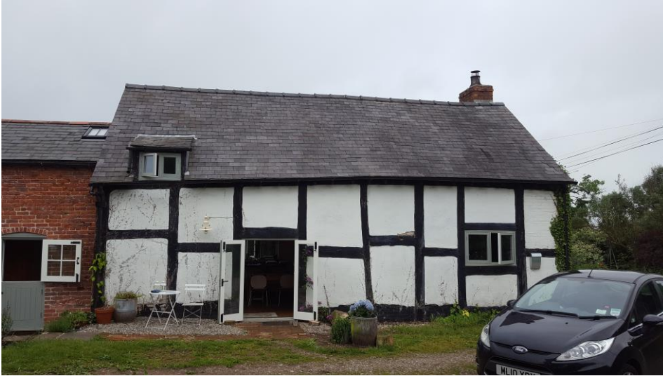
Figure 3 – View looking West towards existing cottage
