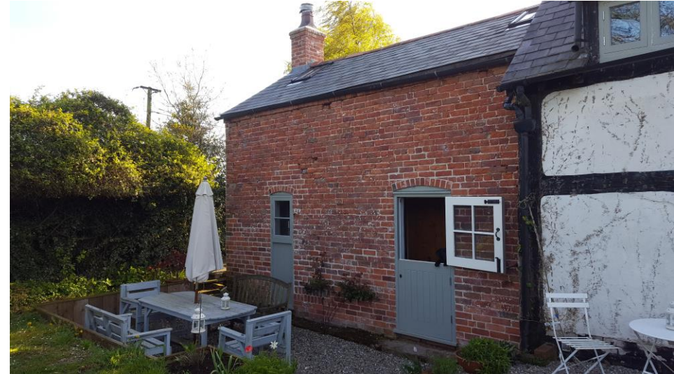
Figure 4 – View looking West towards previously built rear extension
