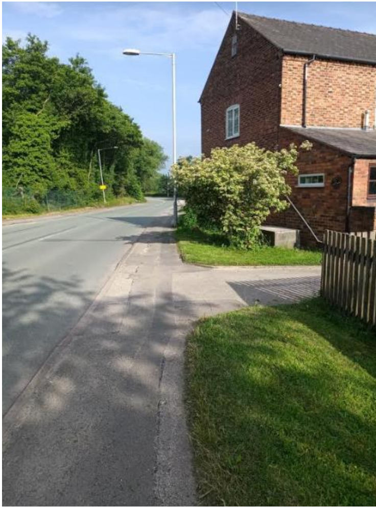
Picture 5: Potential Hazard related to existing access – masked by my house
