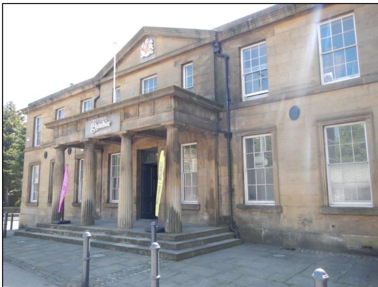
Figure 8: Building B01 (southern elevation)
