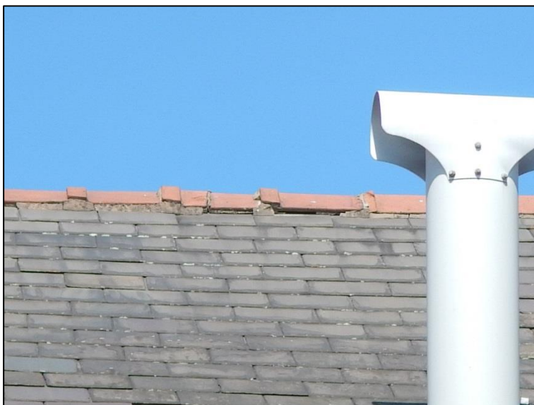
Figure 9: Building B01 (slipped ridge tile)
