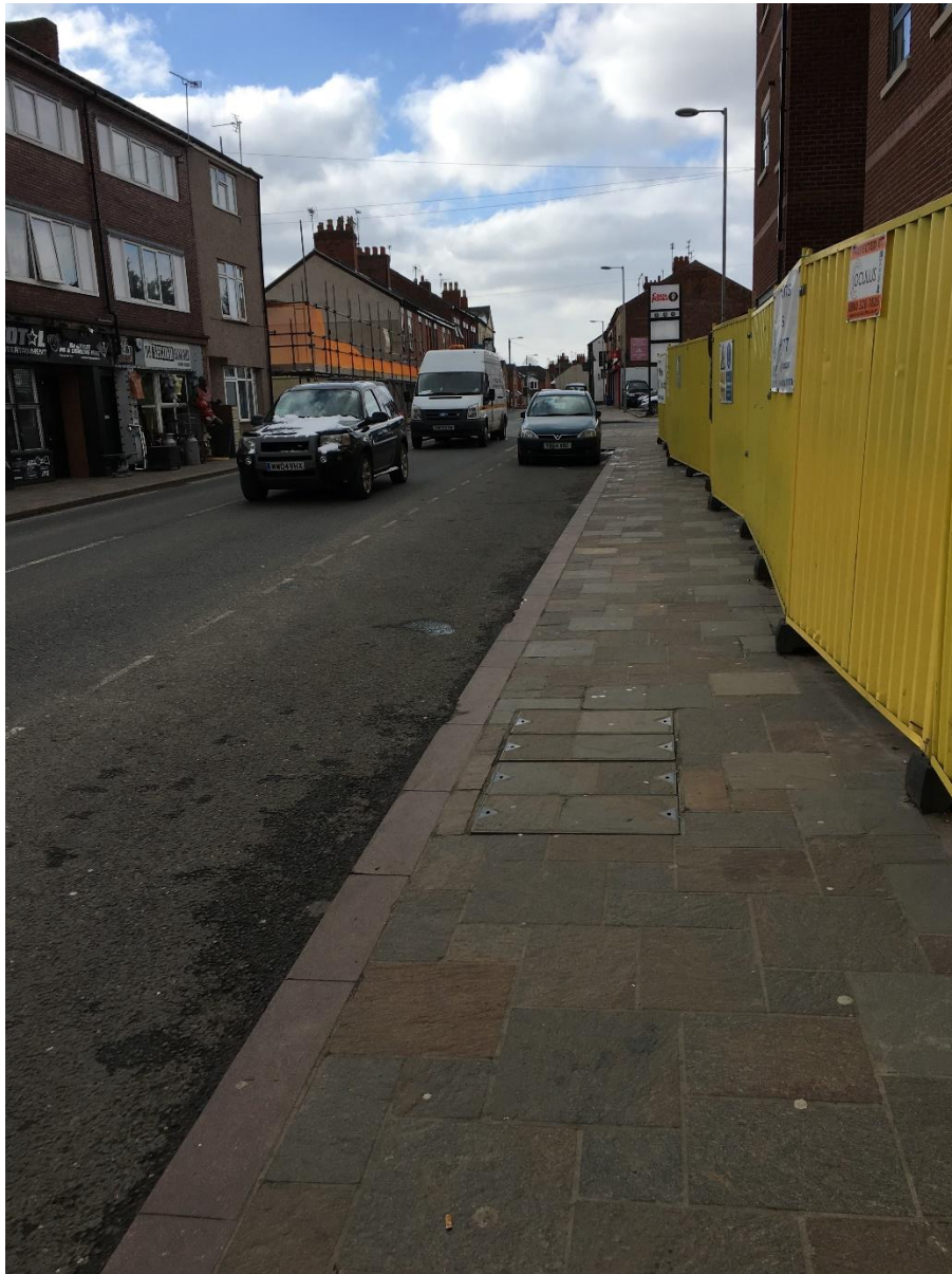
On street parking bays on Bridge Street
