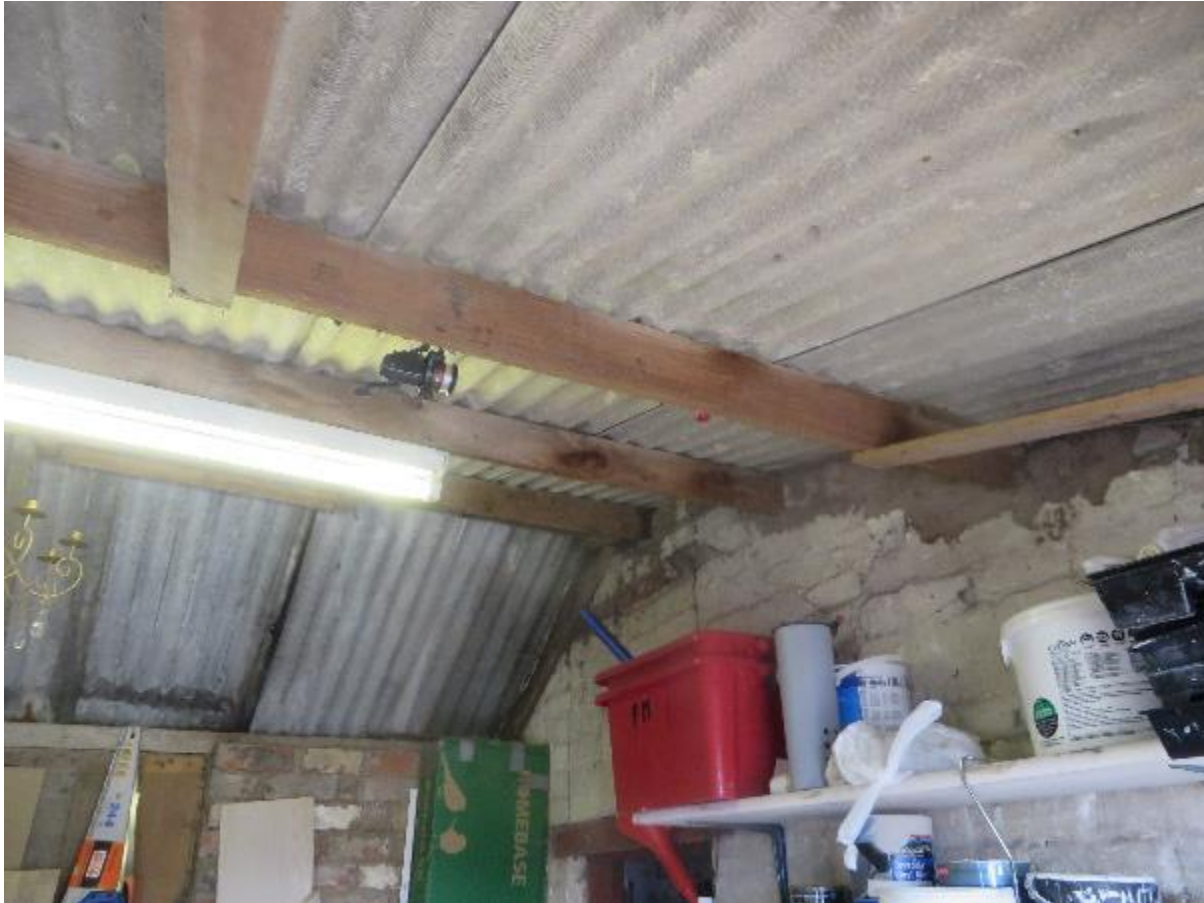
Image 3.14 Typical view inside B1/ S2
