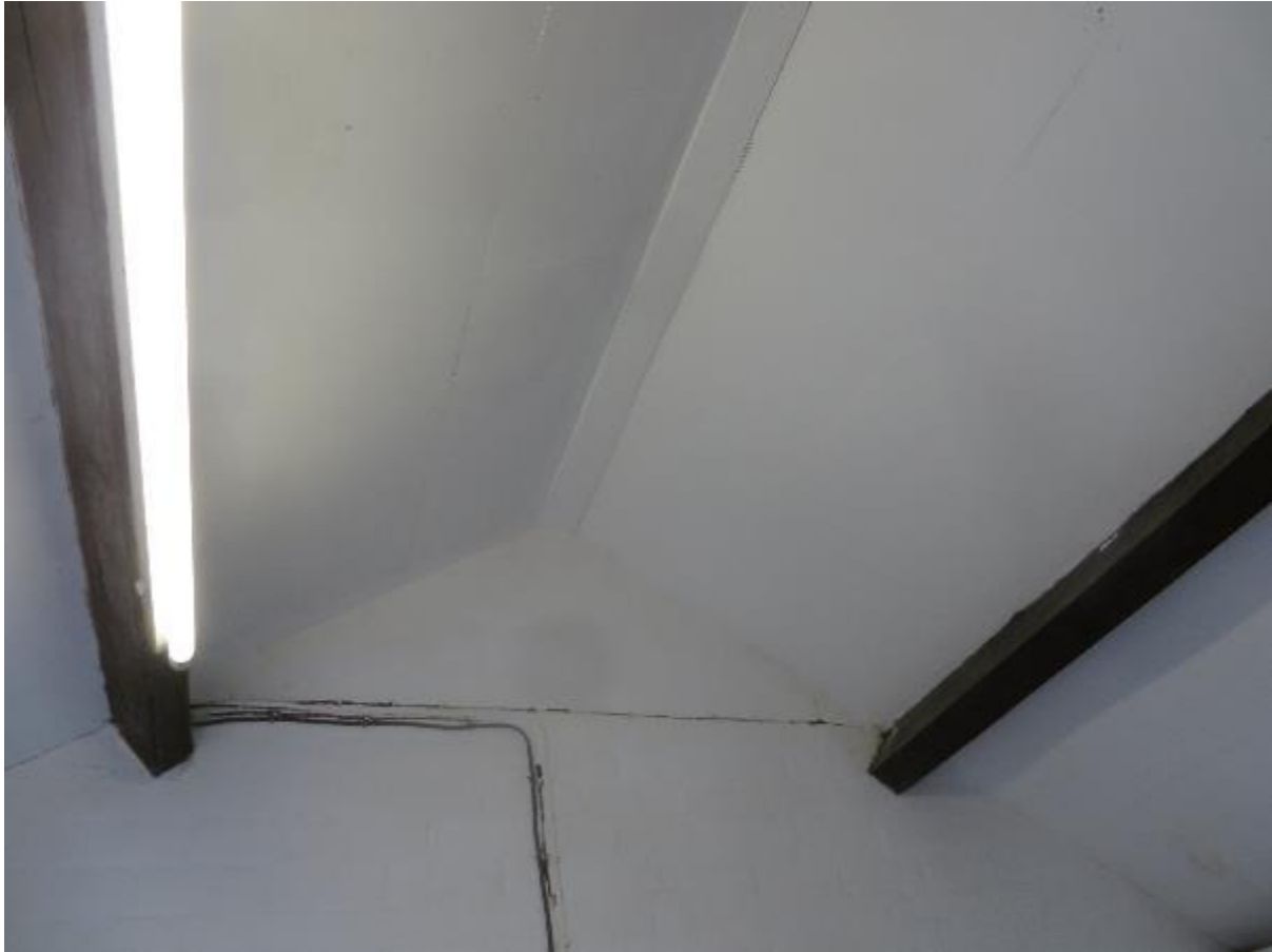
Image 3.12 Open and lit roof space inside B1/ S1
