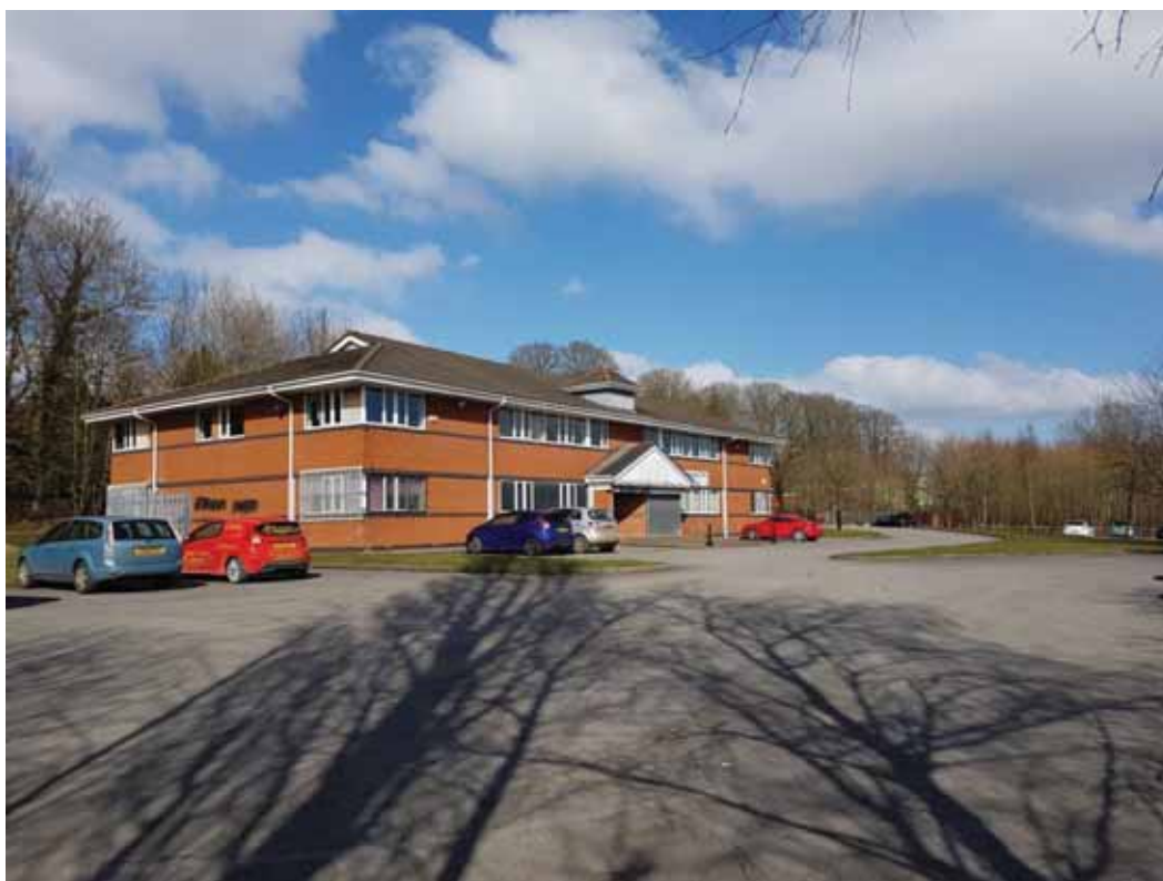
Photographs 1: Main building on site, looking north-westerly.
