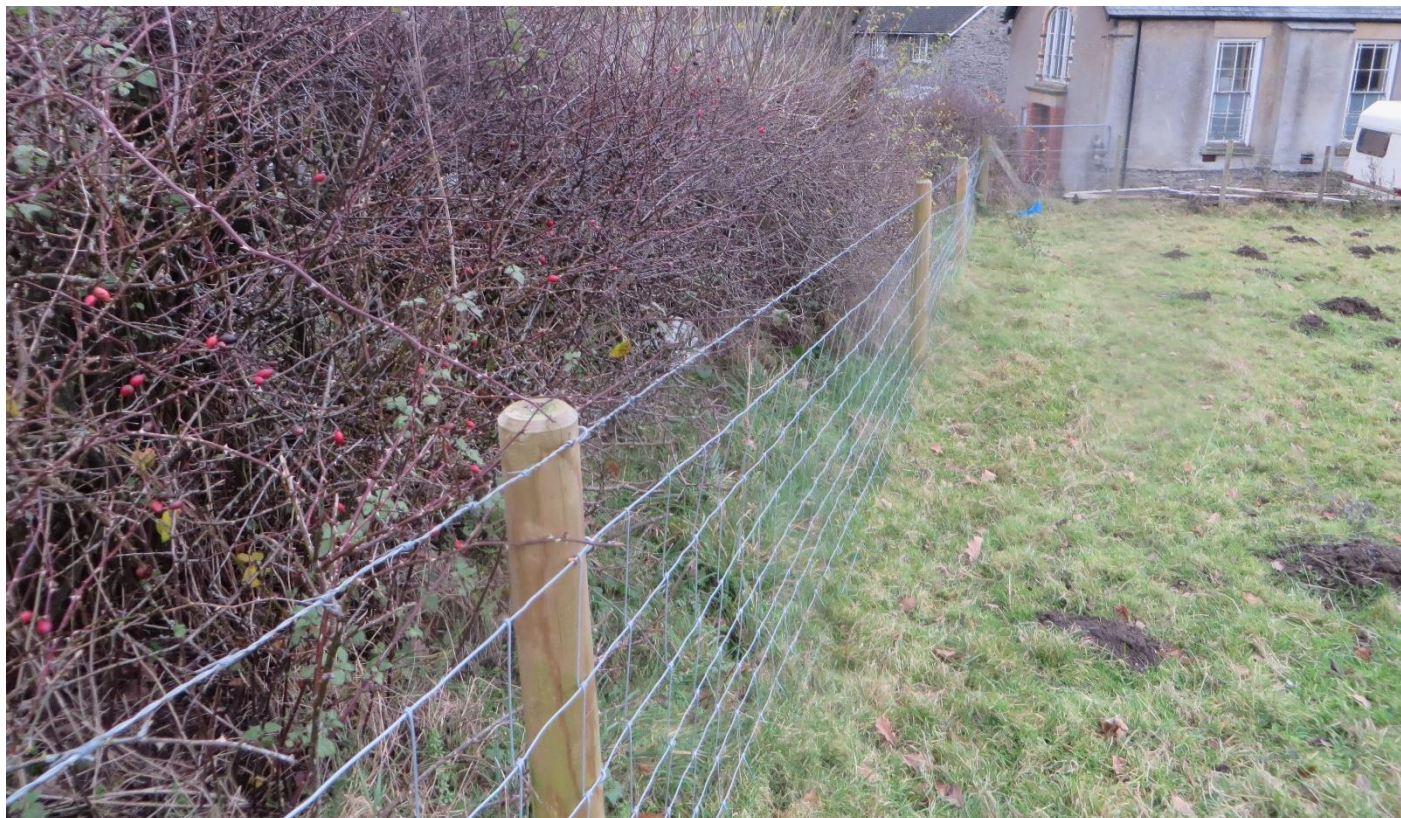
Image 3.6 Moribund hedgerow beyond a post and wire fence along the eastern boundary
