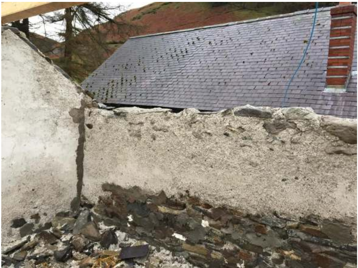
Photograph 6: The east wall from first floor level.
