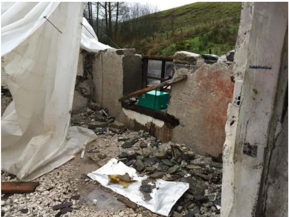
Photograph 10: The west elevation from first floor level.
