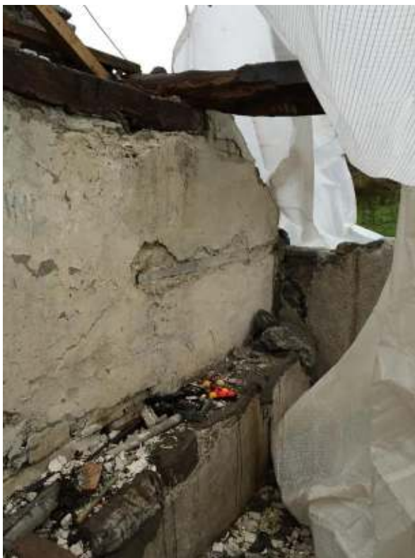
Photograph 2: The south gable viewed from first floor level.
