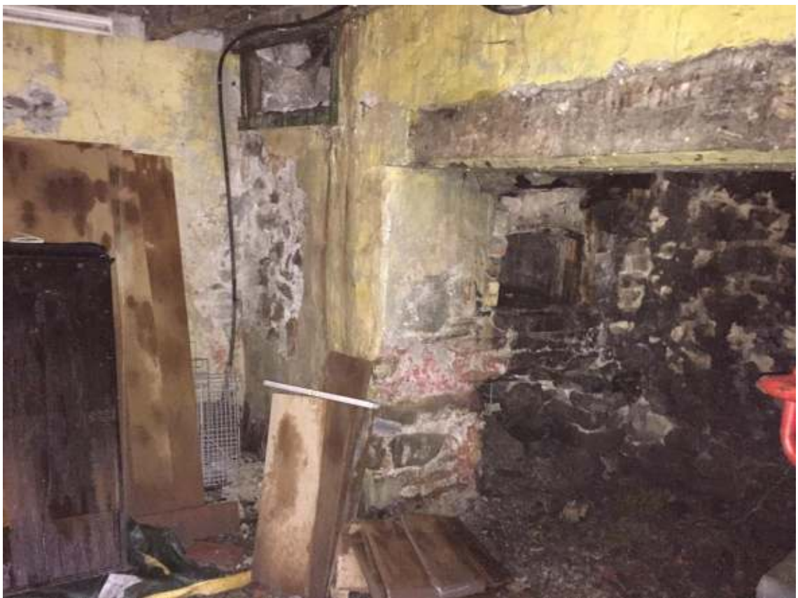
Photograph 13: The fireplace and oven to the south room, ground floor.
