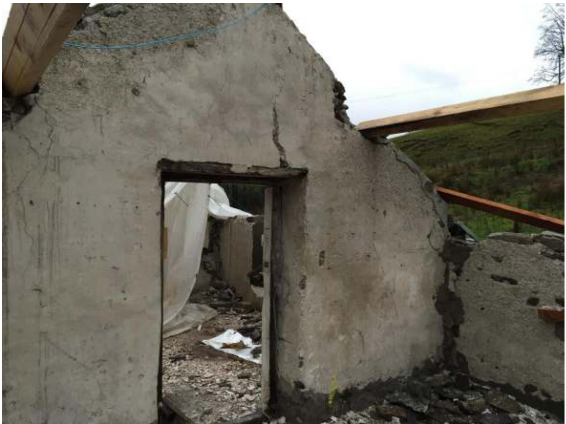
Photograph 8: The central partition first floor looking south west.
