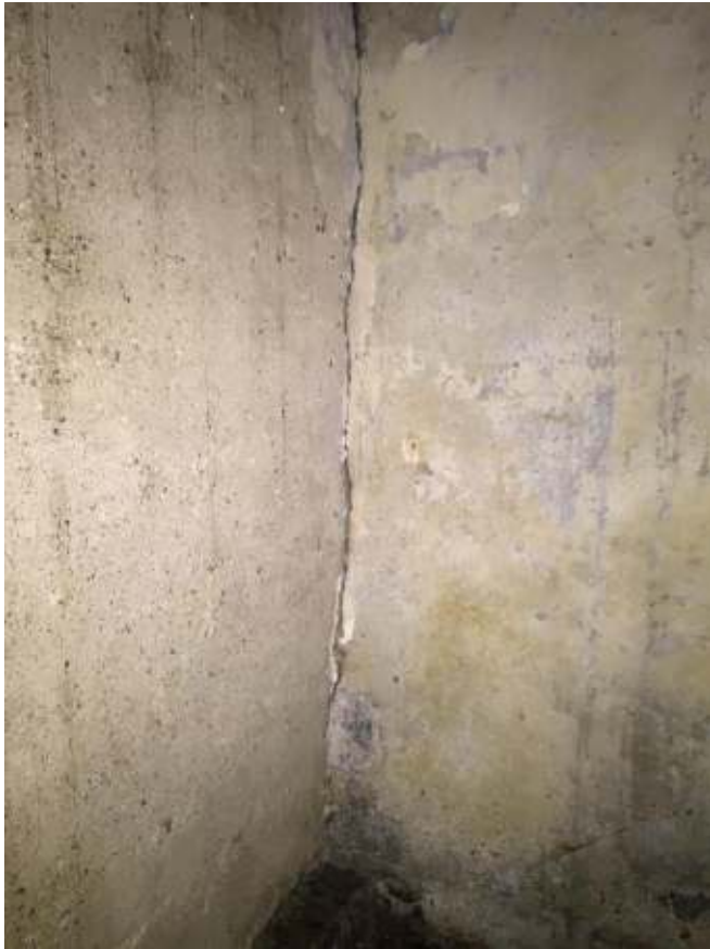
Photograph 17: North east corner of the north room.
