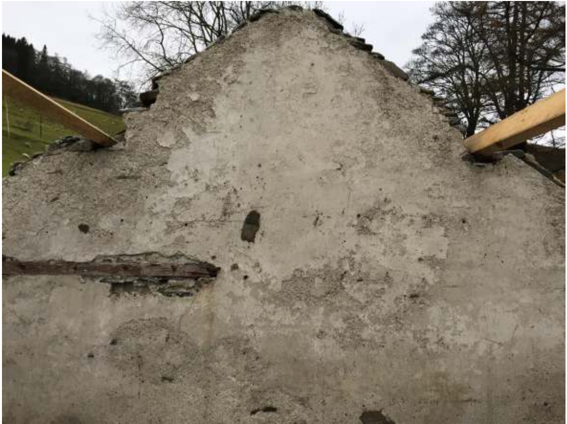
Photograph 5: The north gable from the first floor.
