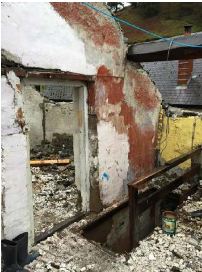
Photograph 4: The central partition first floor looking north east.
