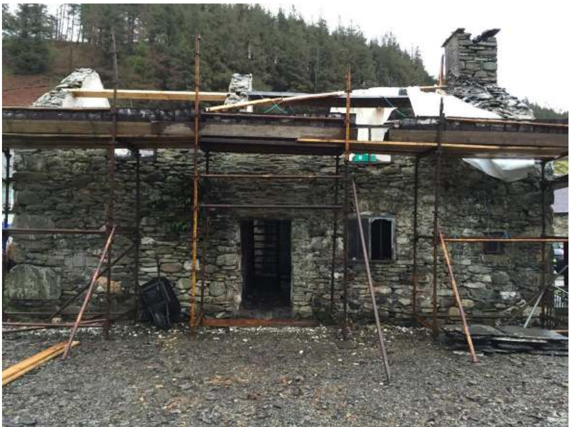
Photograph 18: The west elevation.
