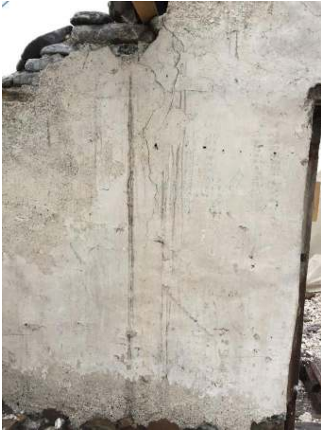
Photograph 9: The central partition first floor looking south.
