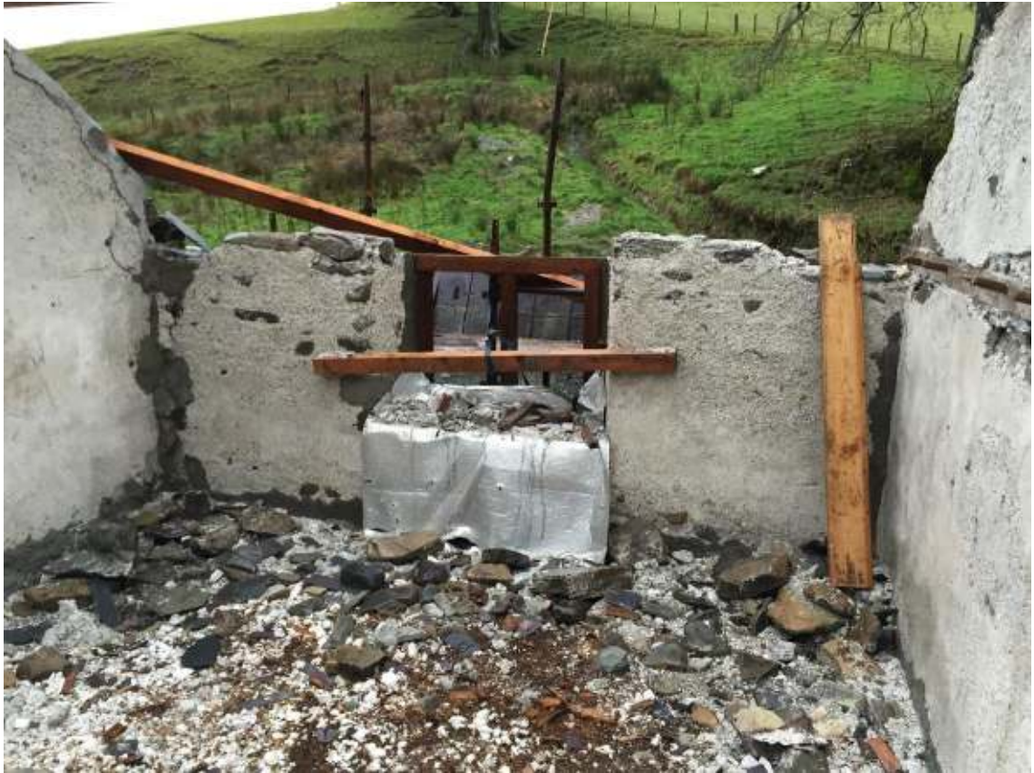
Photograph 7: The west wall from first floor.
