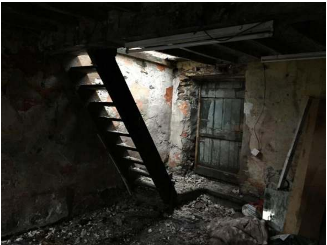
Photograph 12: View from ground floor south room looking north east.
