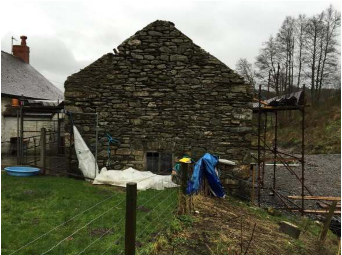
Photograph 19: View of the north gable.
