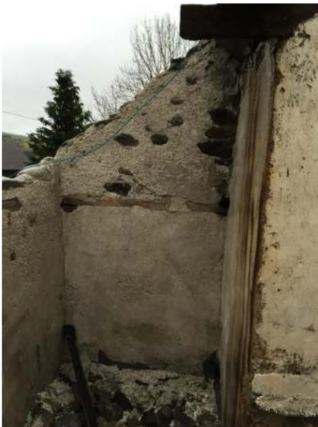
Photograph 3: The south gable viewed from first floor level.
