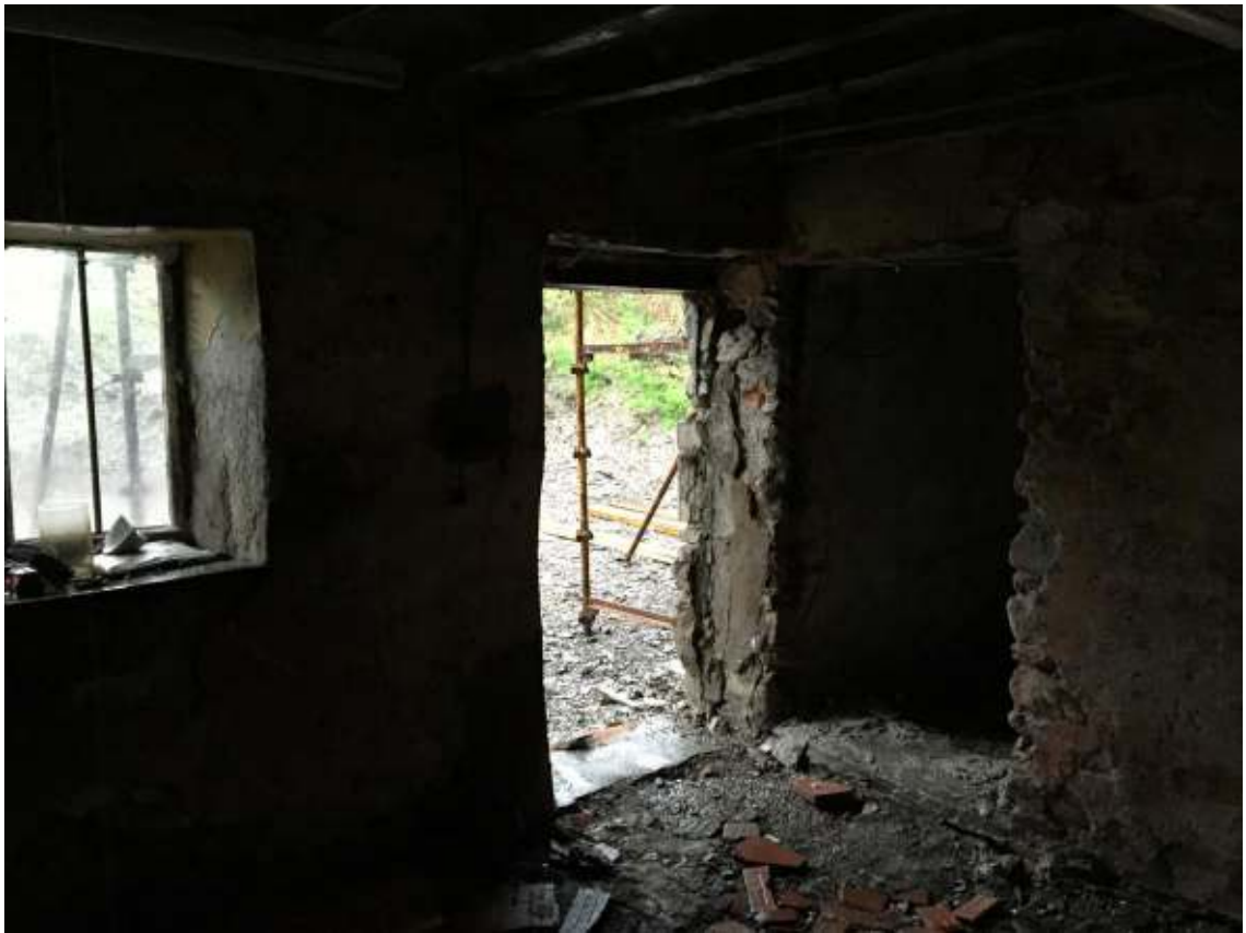
Photograph 11: View from ground floor south room looking west.
