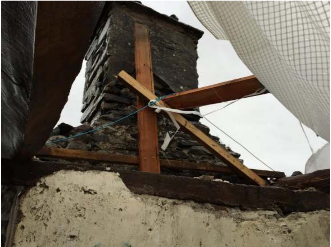
Photograph 1: The chimney stack to the south gable.
