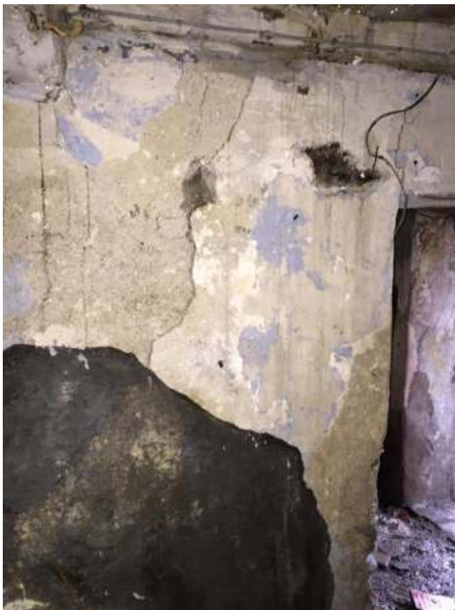
Photograph 16: The partition wall from the north room looking south.
