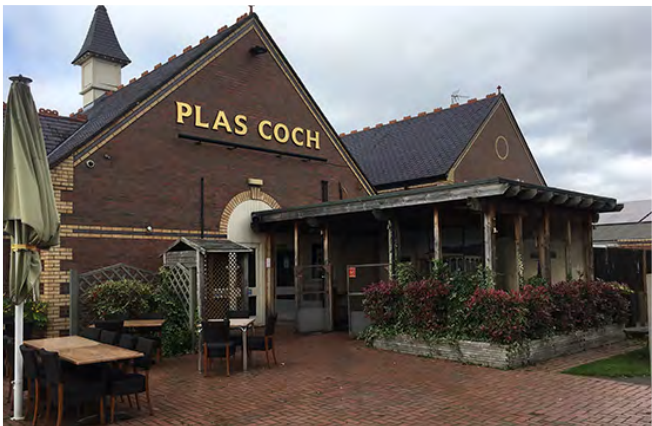
6 - View of the existing pub/restaurant east elevation and the access door for the direct link to the new lodge building.
