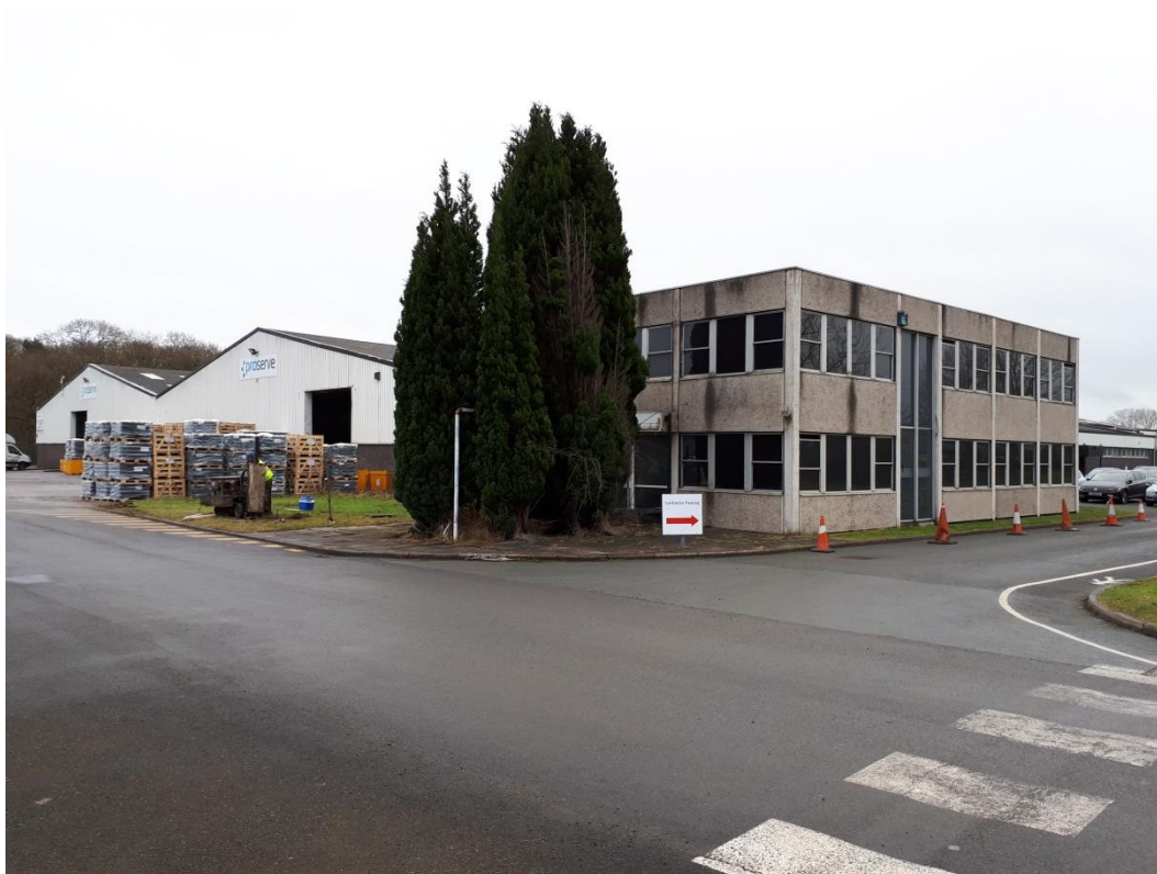
Photograph 1 – From site entrance looking towards the existing buildings
