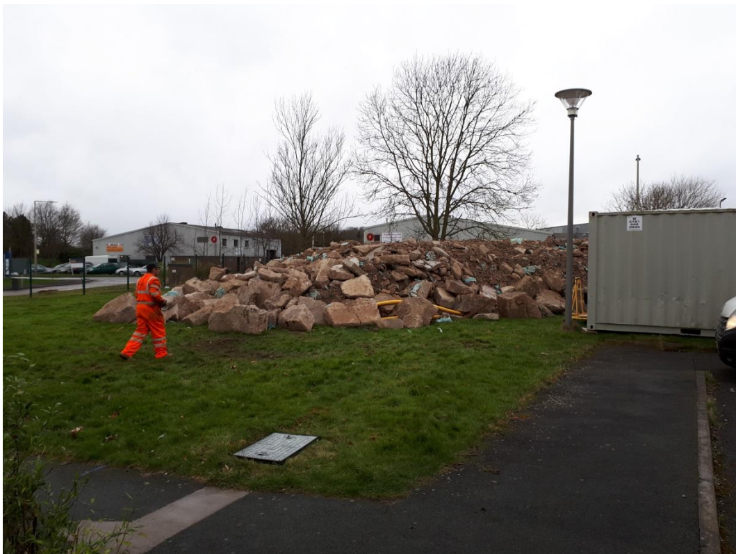
Photograph 4 – South of the industrial unit looking west (stockpile of concrete)
