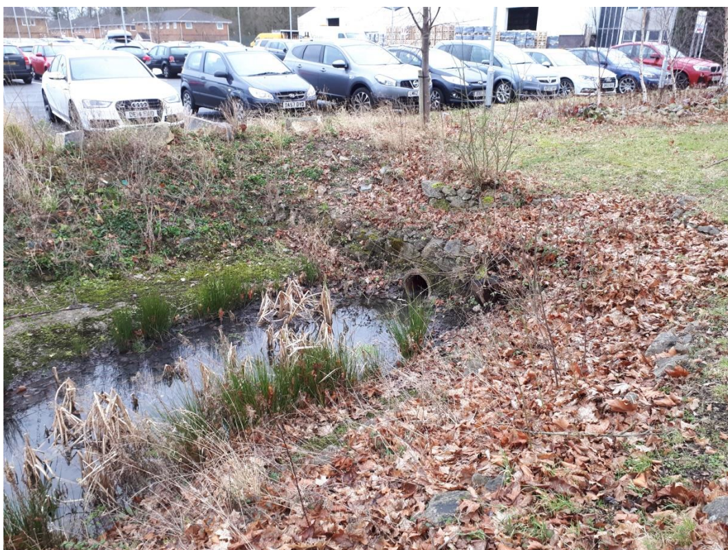
Photograph 8 – Drainage discharge in north west corner of the site
