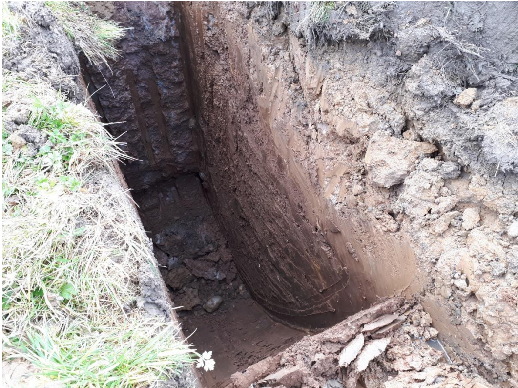
Trial Pit 04 – Pit Walls
