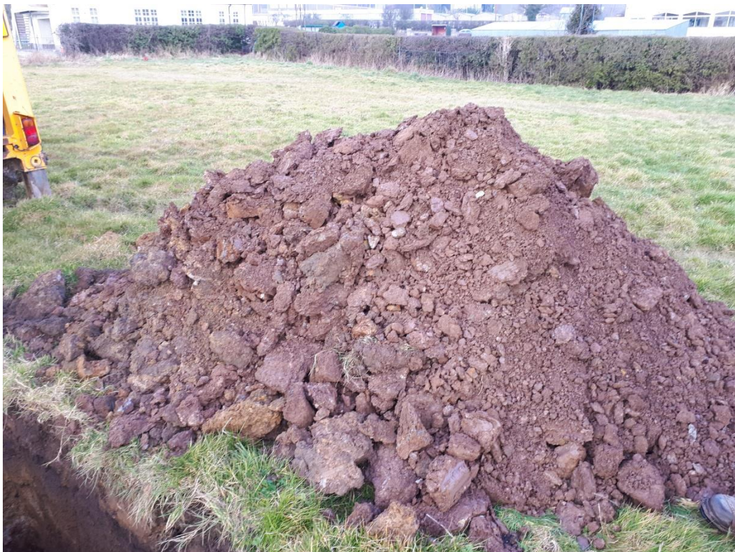
Trial Pit 03 - Arisings
