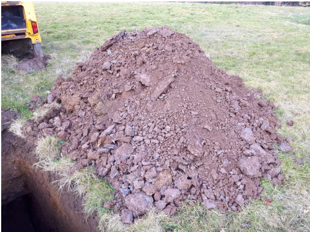
Trial Pit 02 - Arisings
